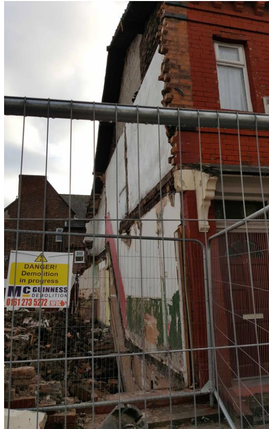
Photograph 5: View facing south of the north western corner of the demolished property and adjoining house.
