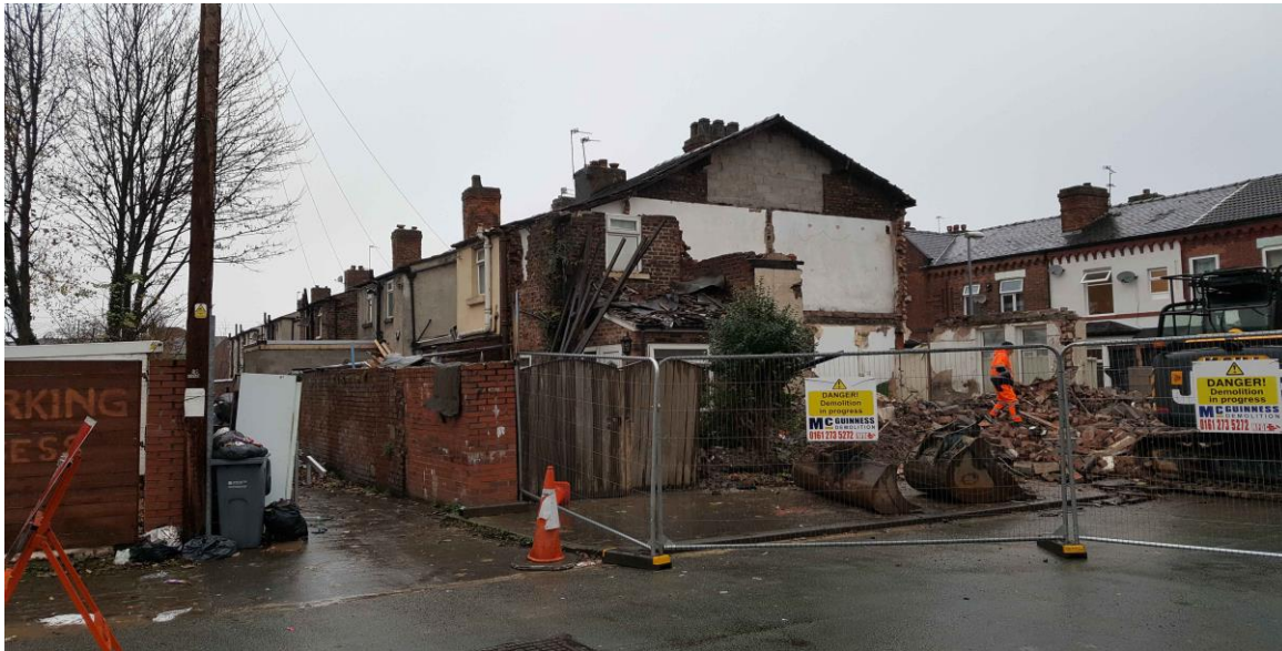
Photograph 3: View facing north west of the demolished property and surrounding area.
