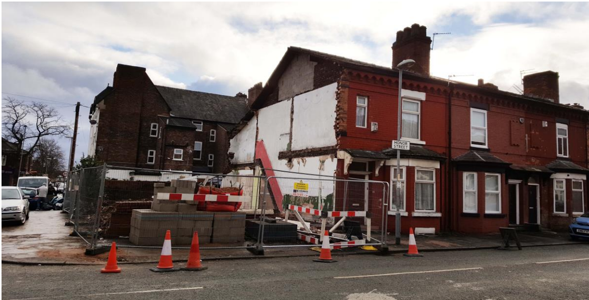
Photograph 1: View facing south of the demolished property
