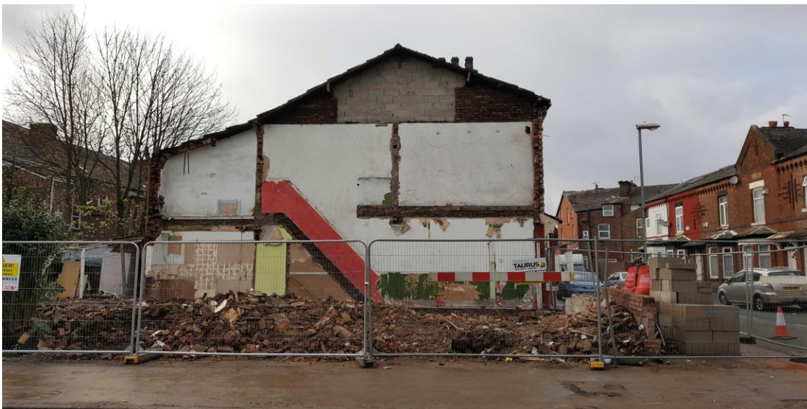
Photograph 2: View facing west of the demolished property
