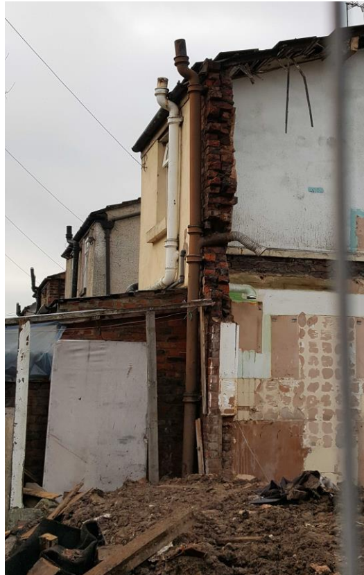
Photograph 4: View facing west of the south western corner of the demolished property and adjoining house.
