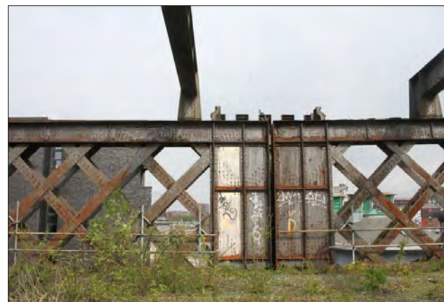
End panels of lattice web spans on the north elevation
