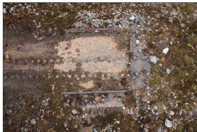
L-section rails rivetted onto deck plate for attachment of longitudinal sleeper
