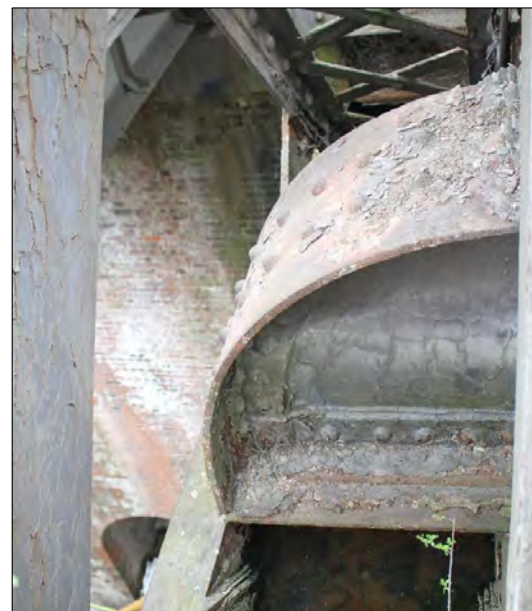
Bull-nosed outer end of fish-bellied transverse girder
