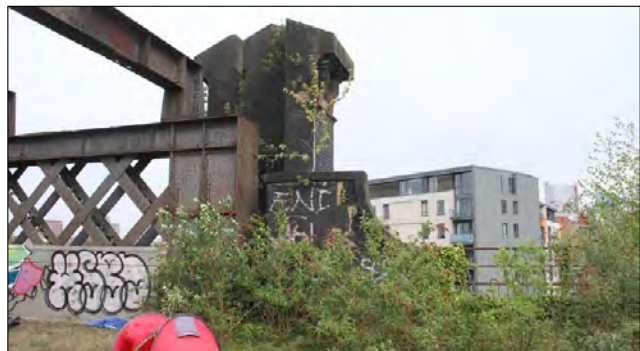
Eastern approach viaduct: north internal face
