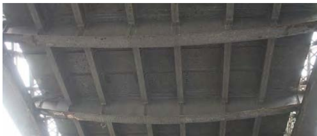
Varying widths of deck plates seen from below
