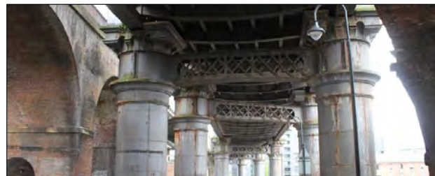
Lattice web Tie Girders spanning between columns across the viaduct
