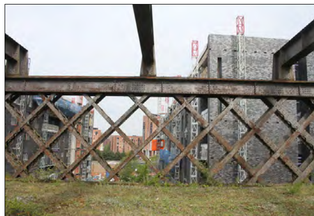
North elevation of lattice web, with reducing thicknesses of lattice bars towards the centre of the span
