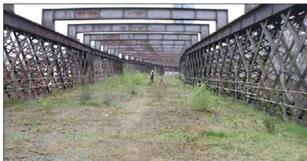
General view of the viaduct looking east, with possible mounding of ballast between the three tracks
