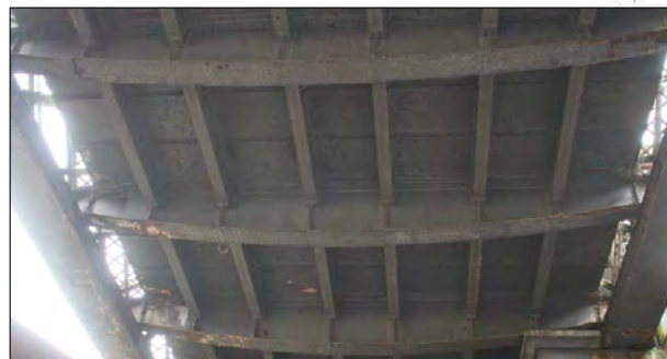
Fish-bellied transverse girders carrying the deck
