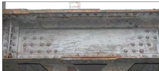
Bracing rail and plates to upper and lower flanges
