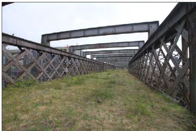
Double-webbed lattice girders forming both sides of the viaduct
