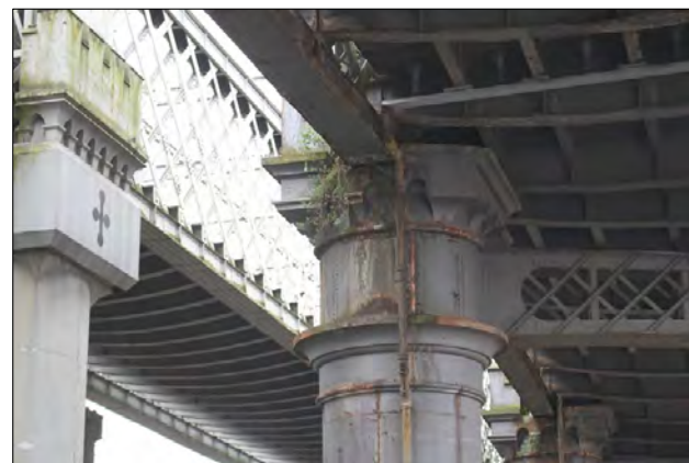
Replaced hoppers and gutter, with original downpipes on the southern columns
