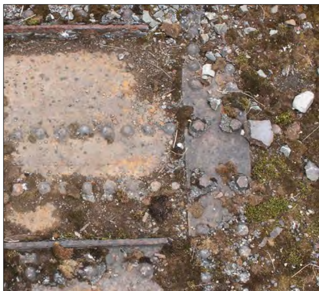
Flat bar with bolts and rivets placed across the deck plates
