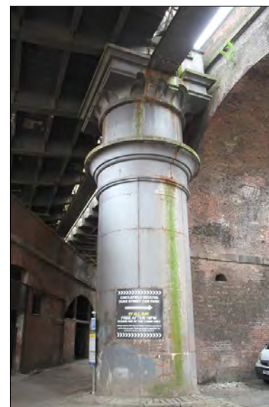
Detail of column
