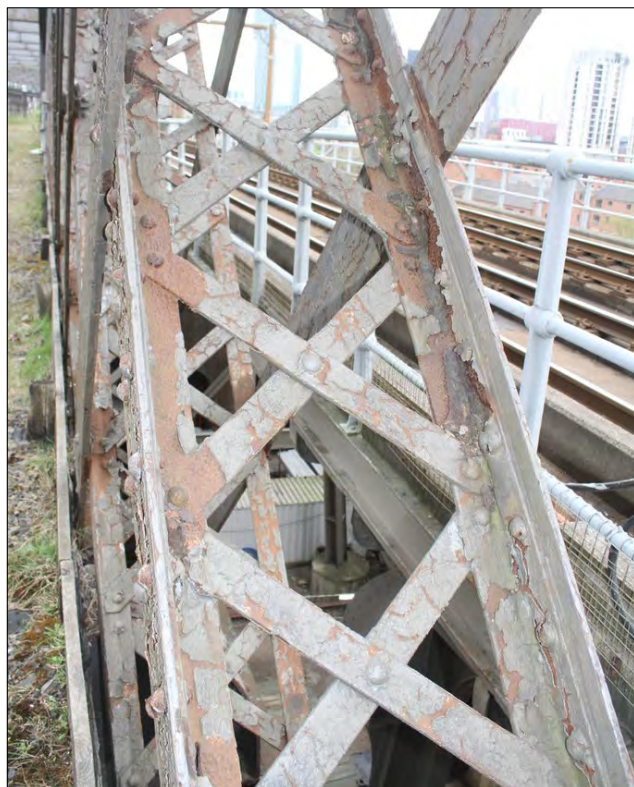
Tie bars (03d) between the two faces of the north elevation, rivetted to L-section rails (03e)
