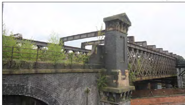
Eastern approach viaduct: detail of decorative pilaster
