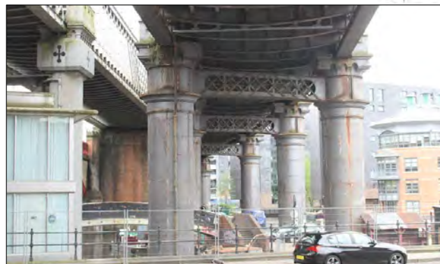
Columns carrying the viaduct
