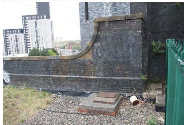
Western approach viaduct: north internal face
