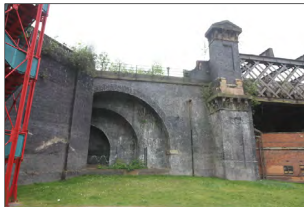
Eastern approach viaduct from the north
