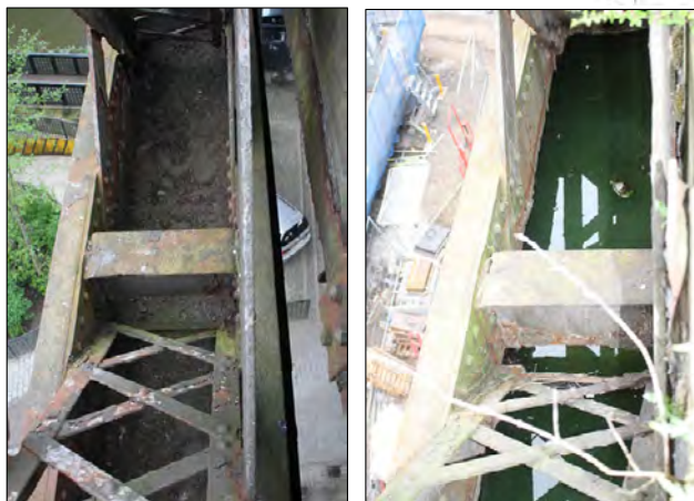
Detail of bottom girder channel, with and without water infilling
