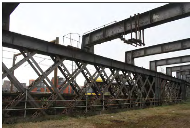
Overhead gantry with access ladder on the southern side of the viaduct
