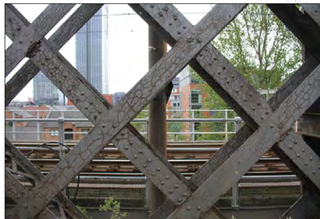
Detail of flat lattice bars
