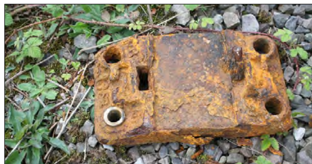
Track baseplate discarded on the deck of the viaduct
