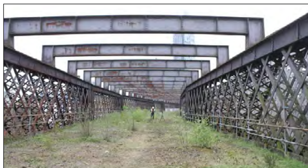
Late steel portal beams that replaced original lattice beams across the viaduct
