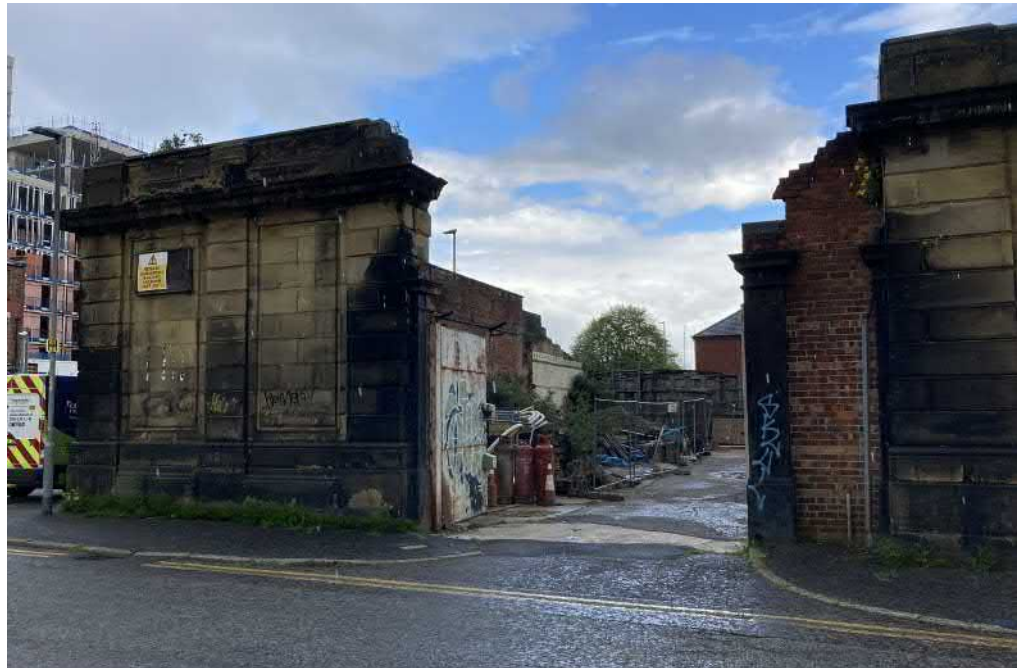
OUTSIDE ELEVATION - WEST END Wall to be partly demolished. East wall corner to be retained and restored.
