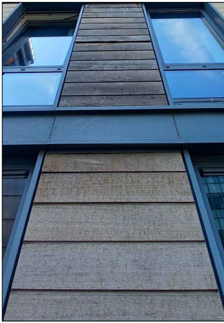
Existing Timber Panels
