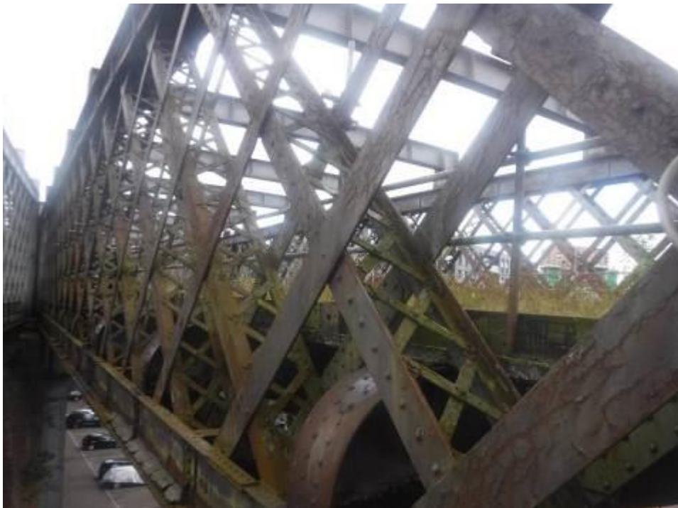
Photograph 139: General view of south truss of span 5
