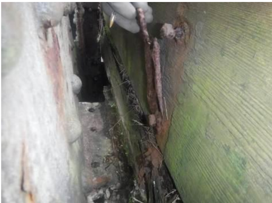
Photograph 232: Typical condition of ballast board fixings to top of deck
