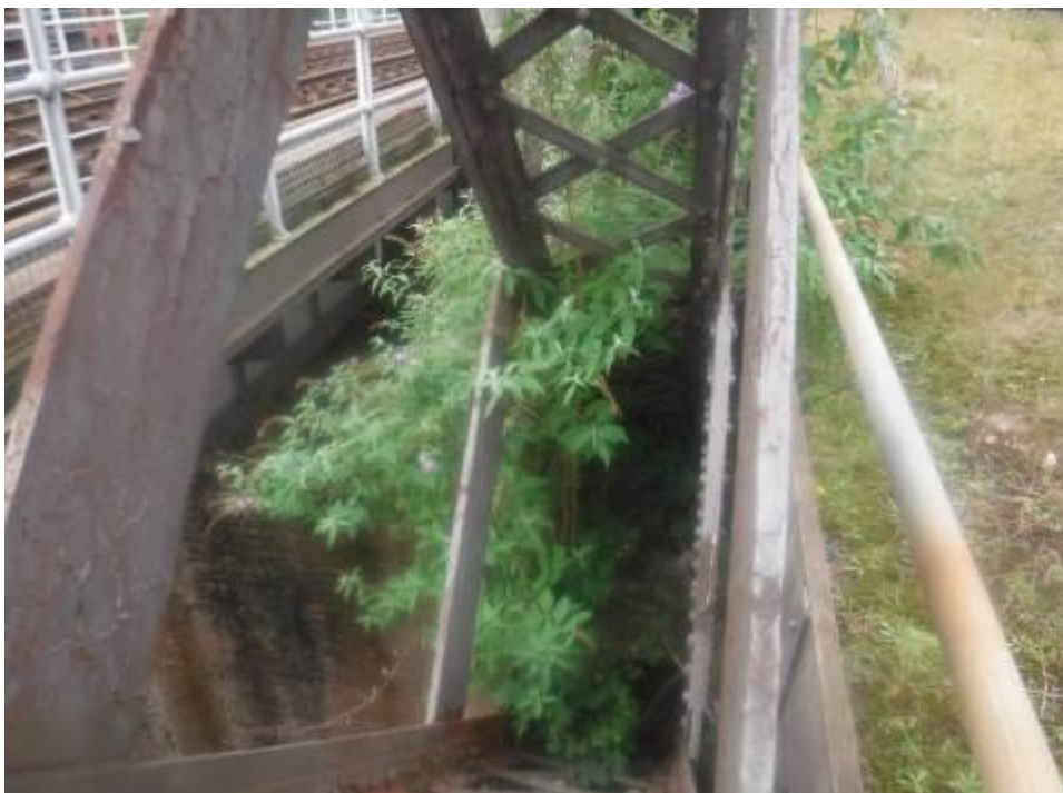
Photograph 161: Loss of thickness & section to end section lowest horizontal stiffener of south truss of span 7
