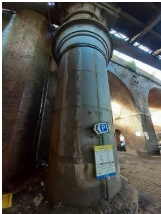
Photograph 38: General view of extra column to span 1
