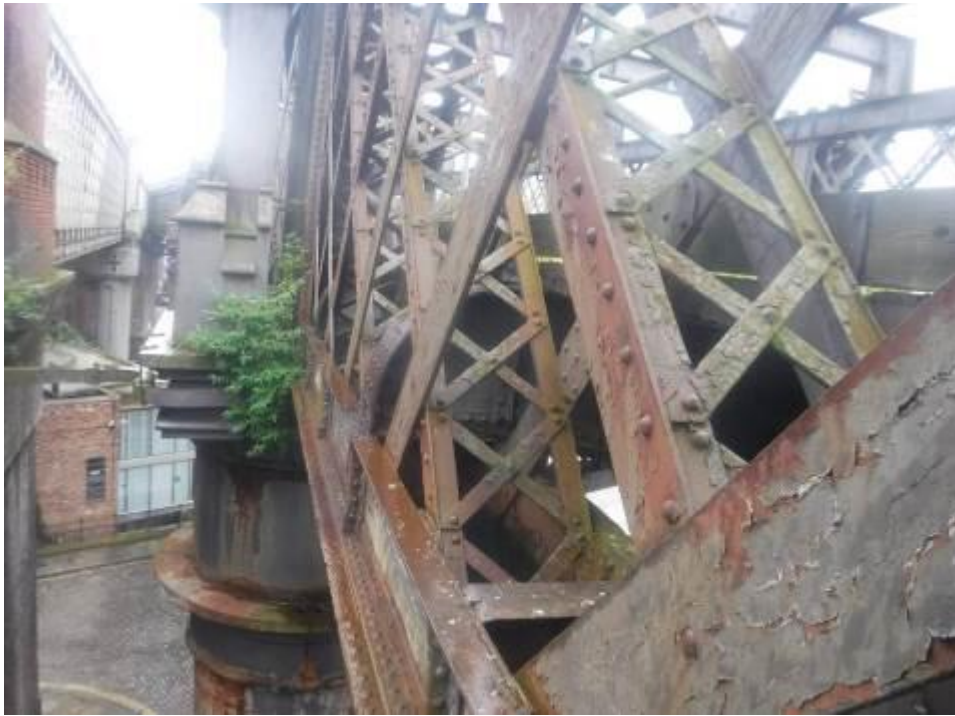
Photograph 107: General view of south truss of span 2
