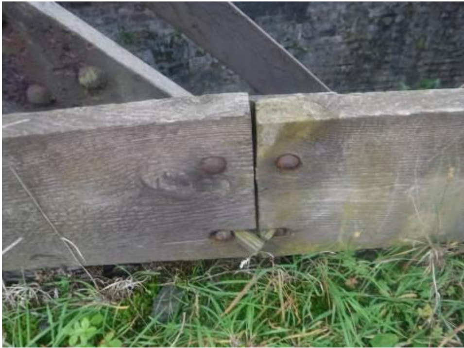
Photograph 231: Typical condition of ballast boards to top of deck
