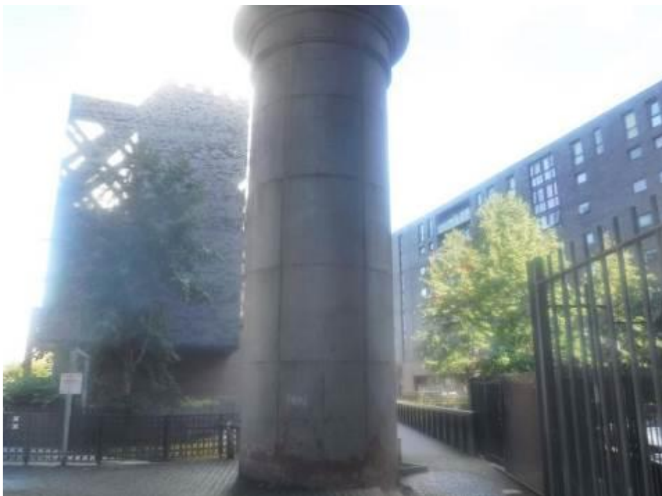
Photograph 80: General view of north column of pier 6
