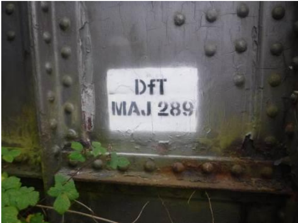
Photograph 11: Parapet structure number
