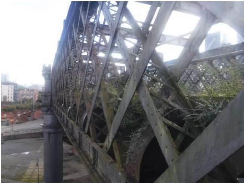
Photograph 131: General view of north truss of span 5
