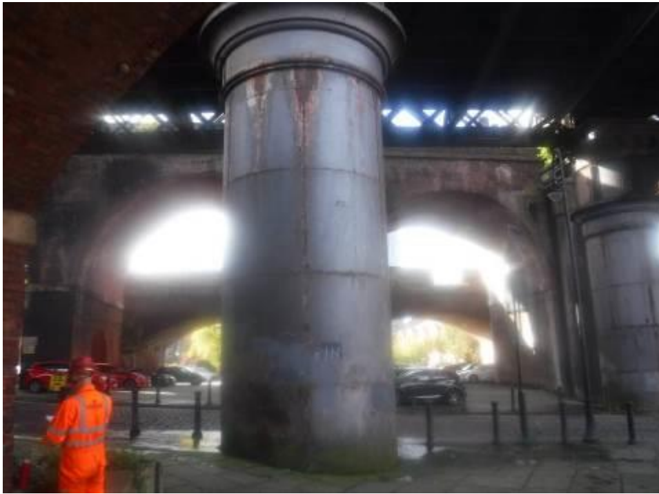
Photograph 35: General view of pier 1, north column
