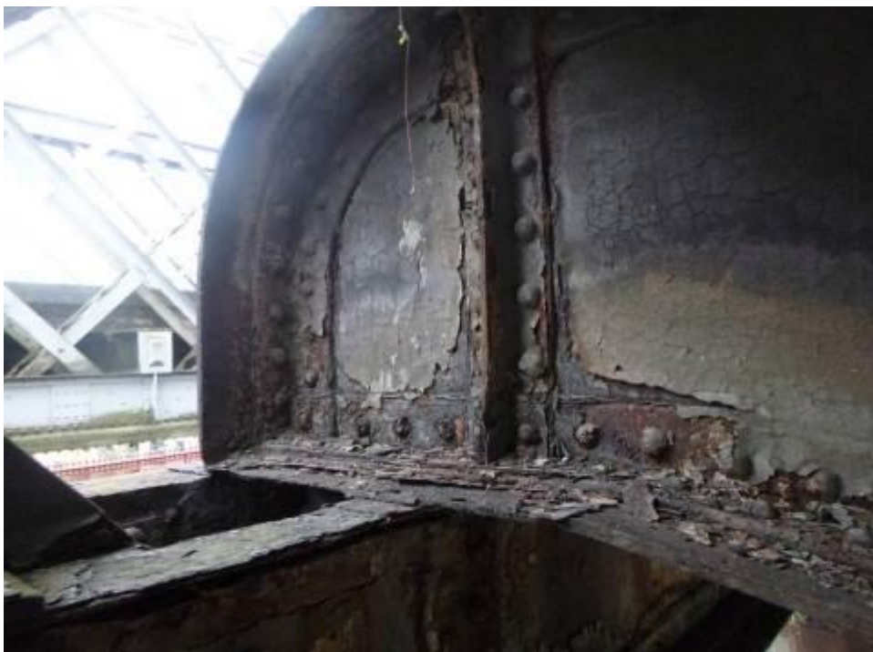
Photograph 194: Typical condition of main / transverse girder connections to soffit of span 4
