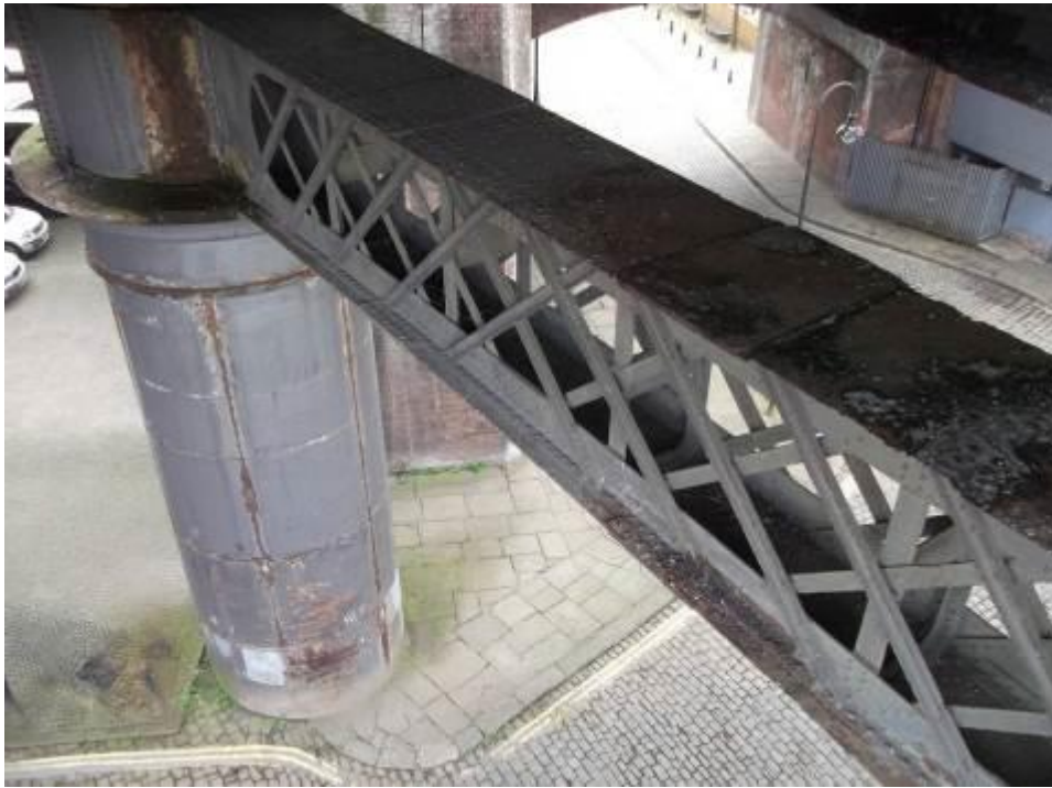
Photograph 45: General view of pier 2, south column and interconnecting truss of pier 2
