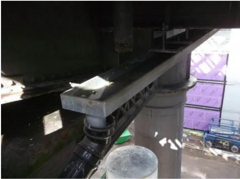
Photograph 211: New gutter system to soffit of span 7
