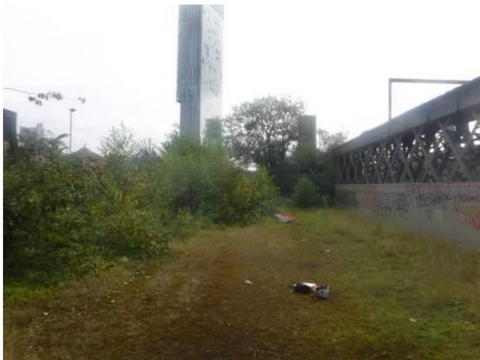
Photograph 5: View from end of structure looking east
