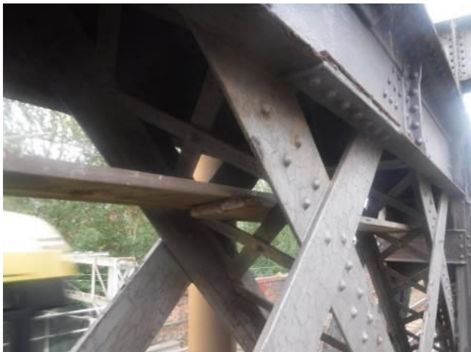
Photograph 171: Scaffold boards to diagonal bracing of south truss of span 8
