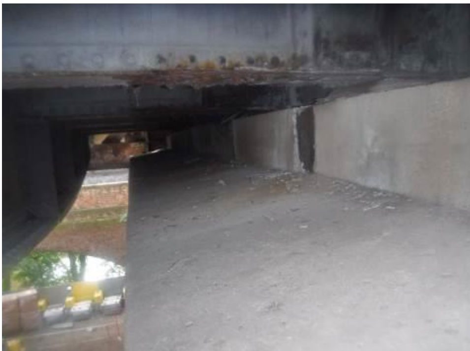
Photograph 20: General view of bearing shelf to west abutment
