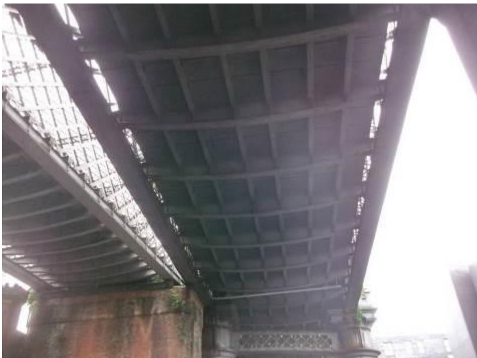
Photograph 200: General view of soffit of span 5
