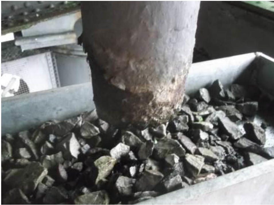
Photograph 201: Ballast to new gutter system of soffit of span 5
