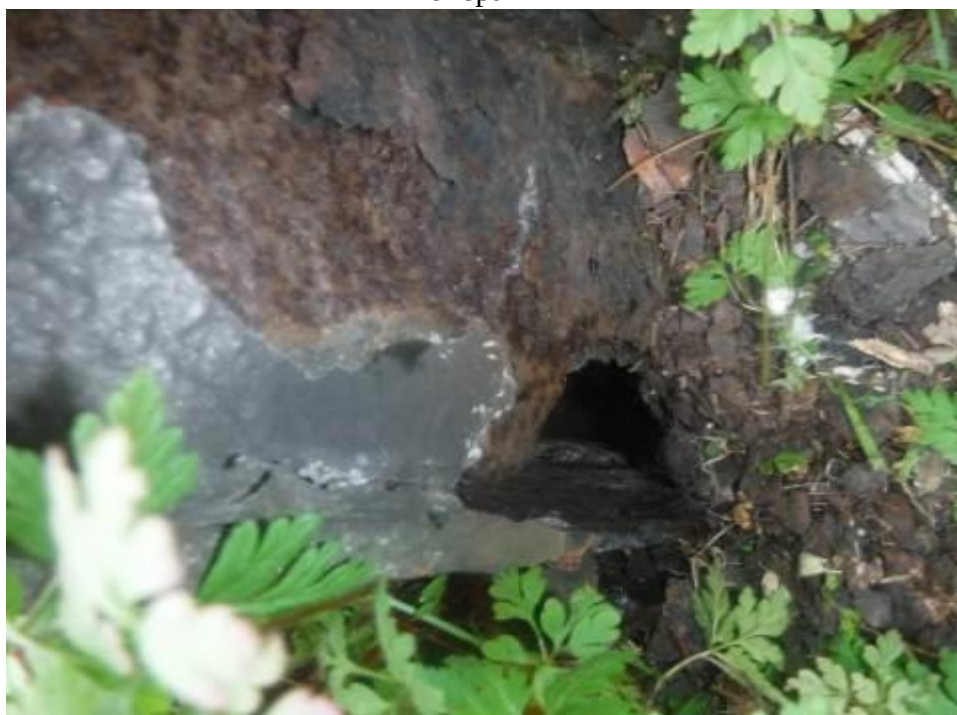
Photograph 157: Typical loss of thickness to bottom boom connections with transverse girders of north truss of span 7
