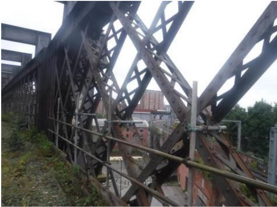
Photograph 99: General view of north truss of span 2
