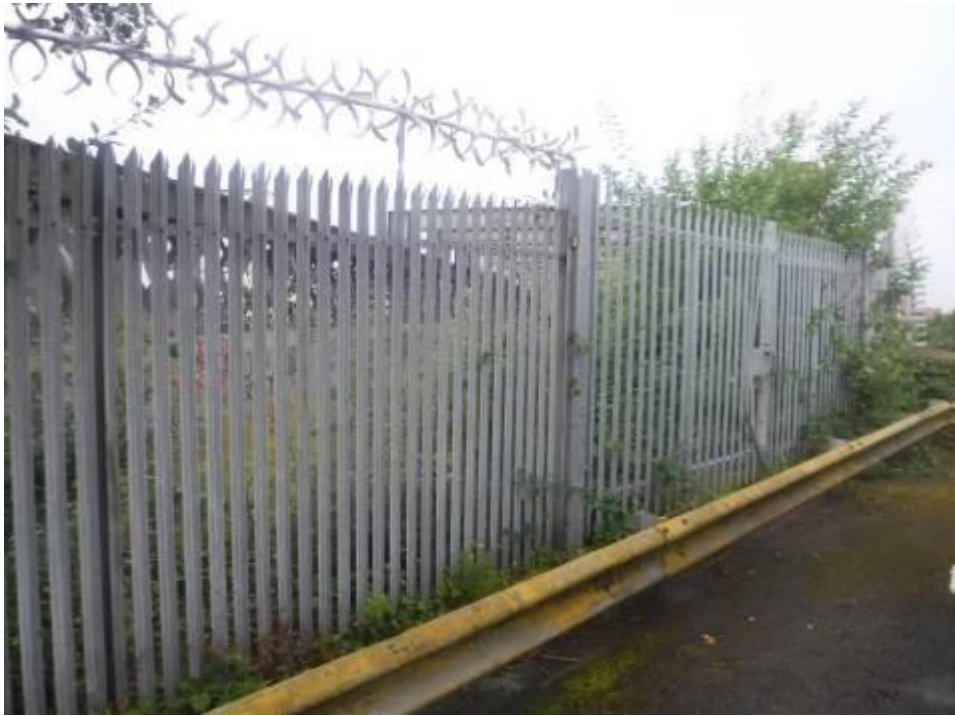
Photograph 7: Palisade fencing to east end
