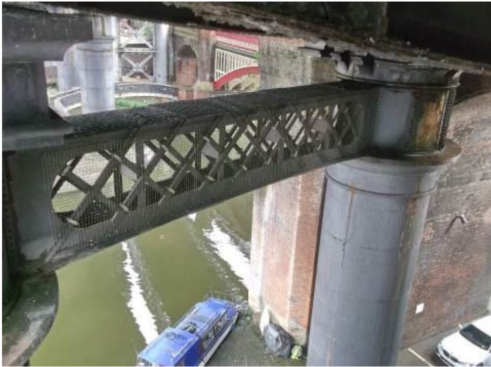
Photograph 77: General view of interconnecting truss of pier 5
