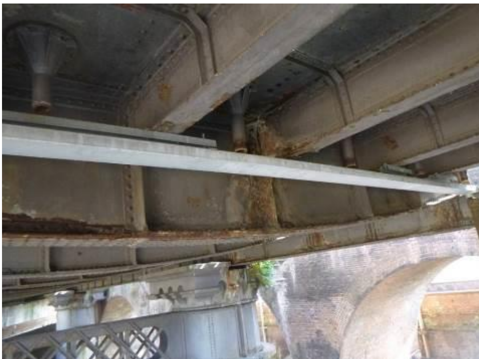
Photograph 180: New gutter system to soffit of span 2
