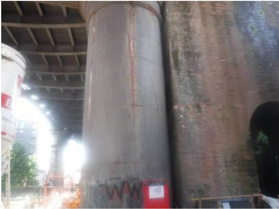
Photograph 83: General view of south column of pier 7
