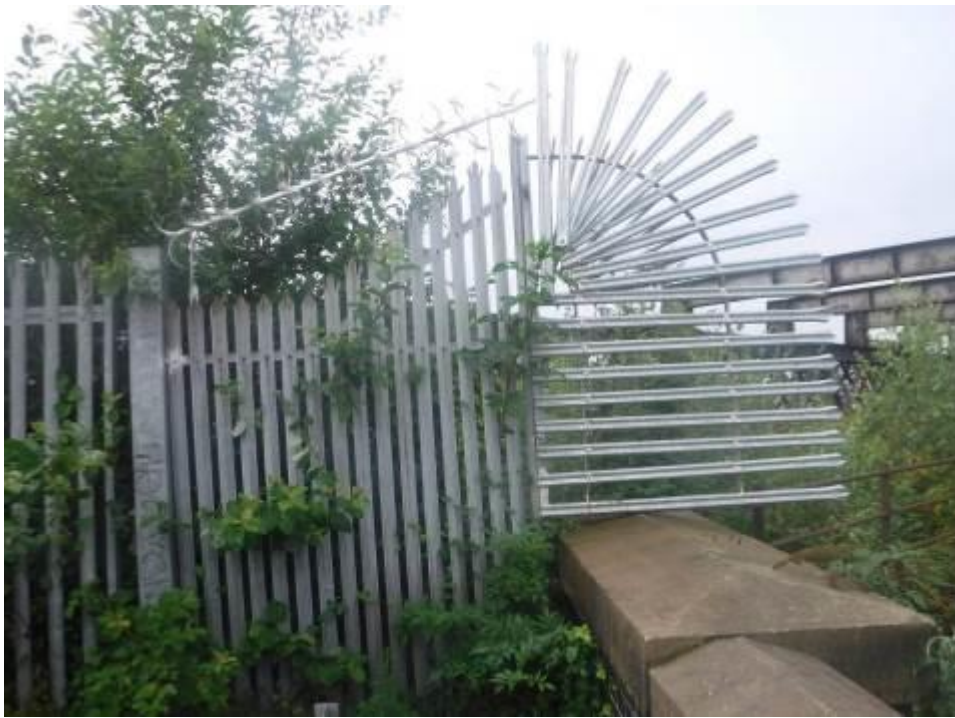
Photograph 239: General view of anti-vandal fencing to top of deck
