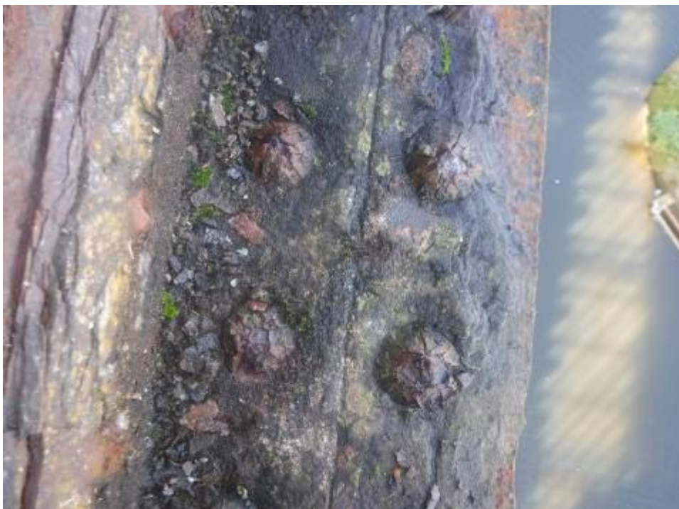
Photograph 132: Typical spiking to lower flange rivets of north truss of span 5
