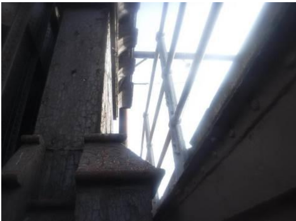
Photograph 92: Typical proximity to Metrolink bridge & OLE of south castle façades to piers
