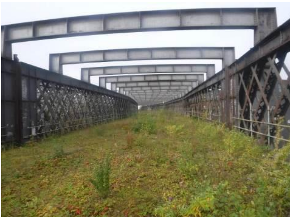
Photograph 4: View along top of structure looking west
