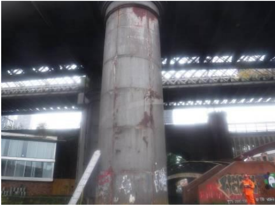
Photograph 53: General view of north column of pier 3
