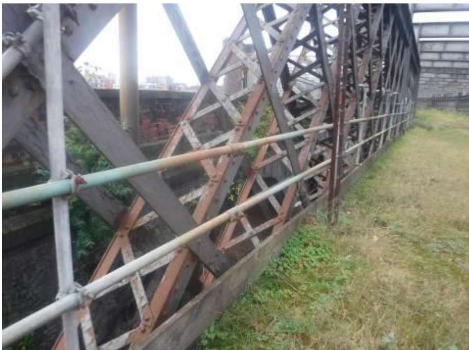
Photograph 230: General view of ballast boards held in place with scaffold bars to top of deck
