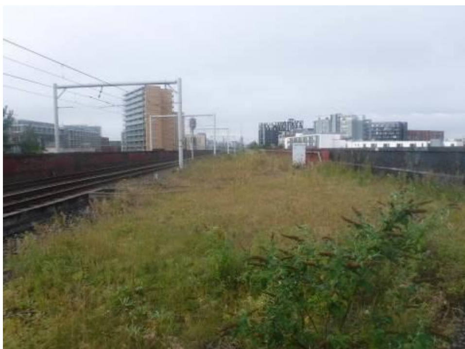
Photograph 6: View from end of structure looking west
