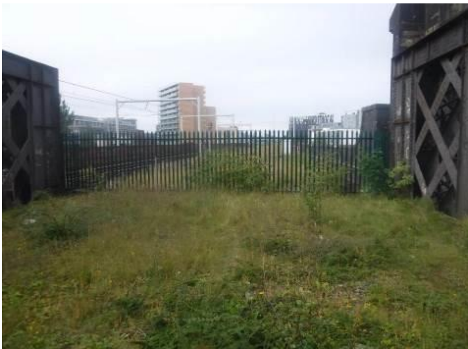
Photograph 8: Palisade fencing to west end
