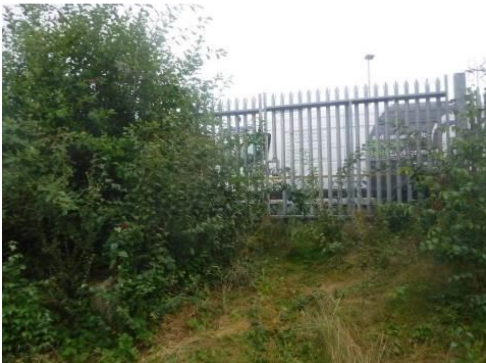
Photograph 228: Typical vegetation growth to top of deck
