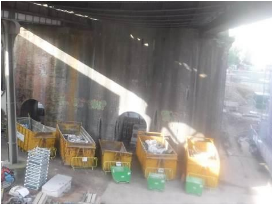
Photograph 19: General view of west abutment
