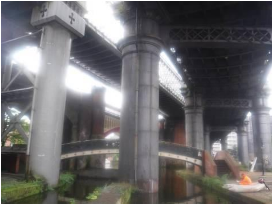
Photograph 55: General view of south column of pier 3
