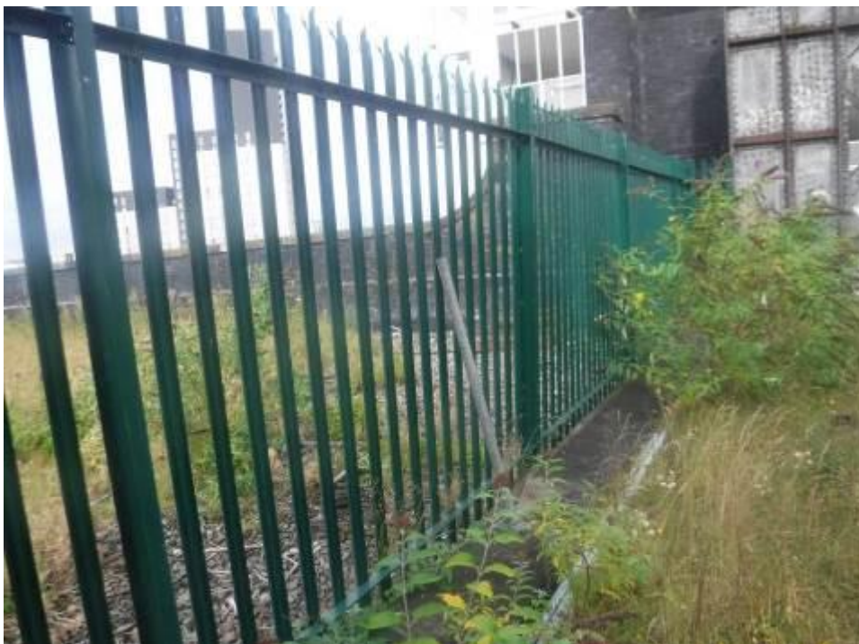
Photograph 240: General view of palisade fencing to west end of top of deck
