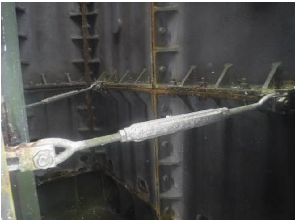
Photograph 94: Typical condition of tie bar connections to castle façades of piers
