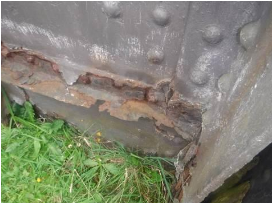
Photograph 161: Loss of thickness & section to end section lowest horizontal stiffener of south truss of span 7
