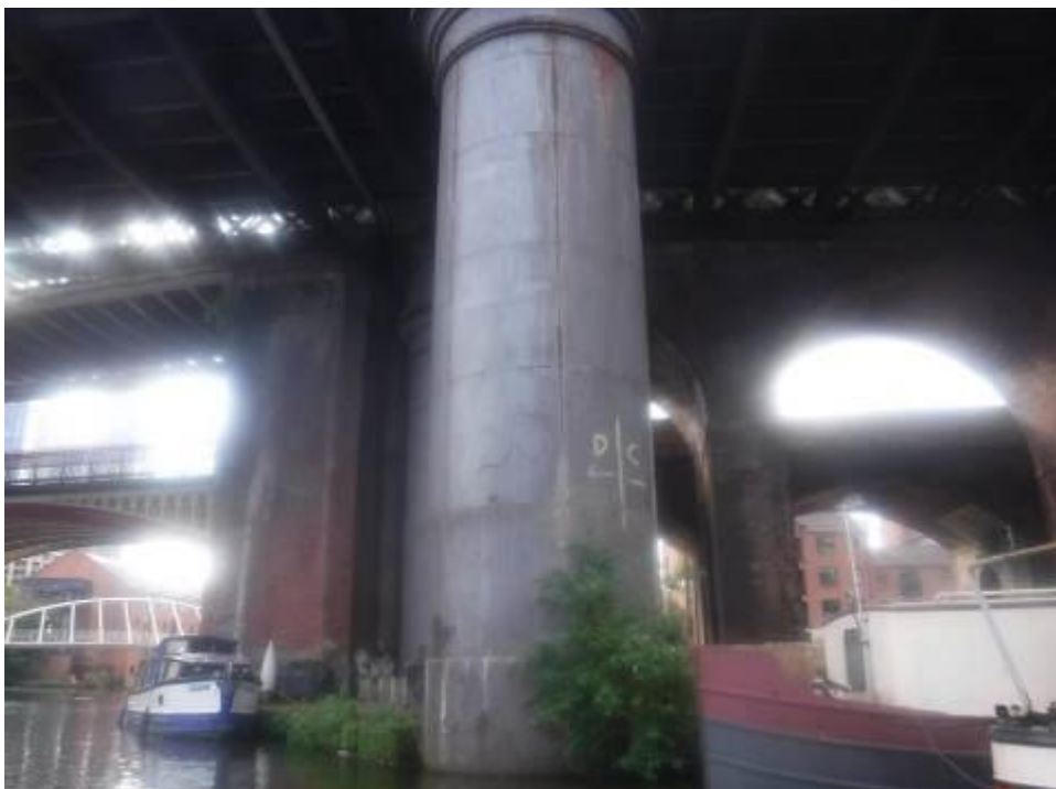
Photograph 76: General view of north column of pier 5
