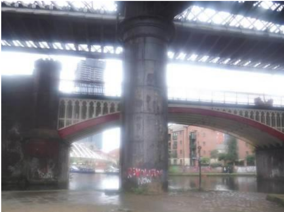
Photograph 63: General view of south column of pier 4
