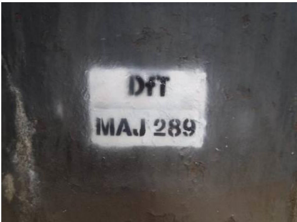
Photograph 12: Pier 1 structure number
