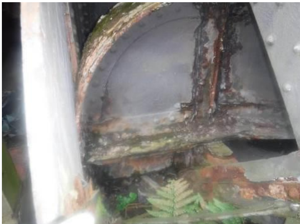
Photograph 157: Typical loss of thickness to bottom boom connections with transverse girders of north truss of span 7
