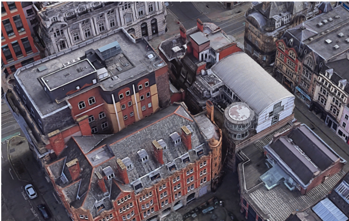
Photograph 15: Google Aerial View of Site (showing existing condensers)
