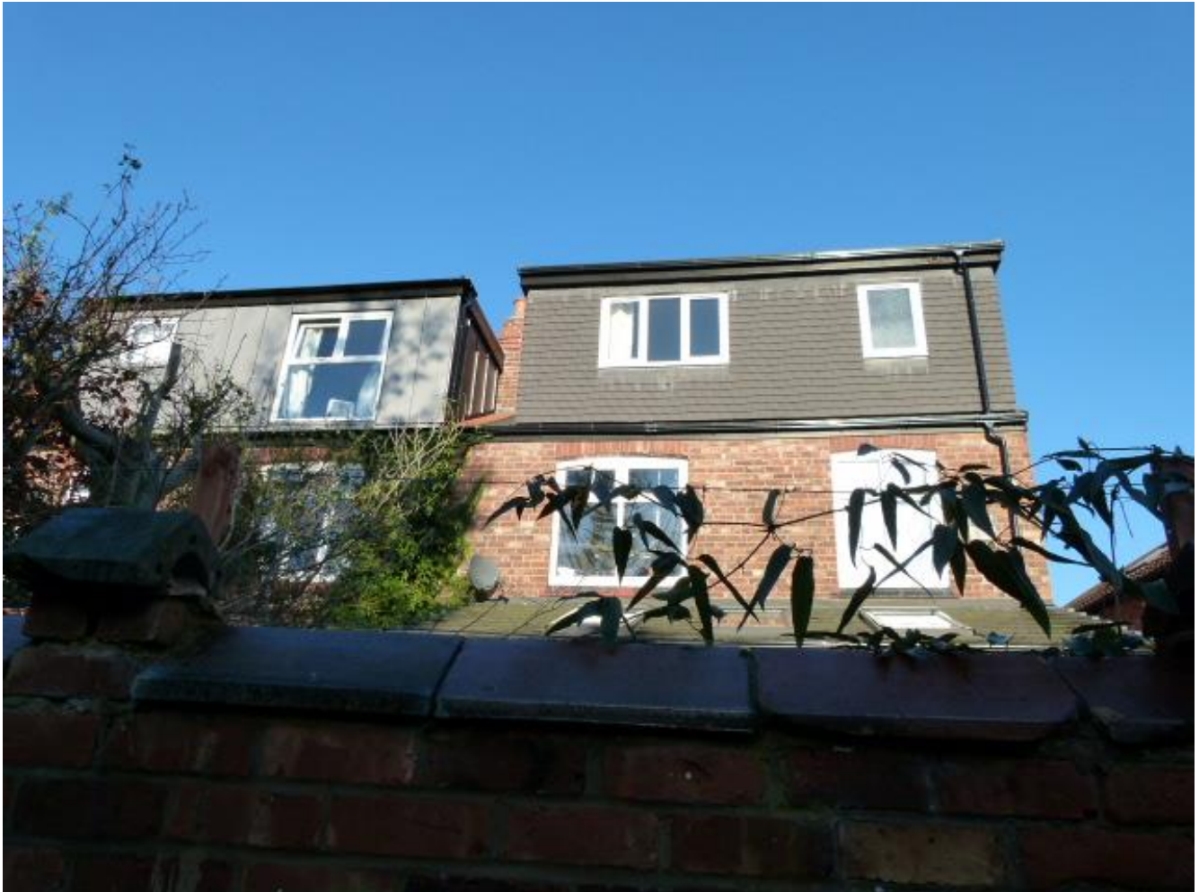
Nos.10 (left) and 12 Gaddum Road to the rear of the site
