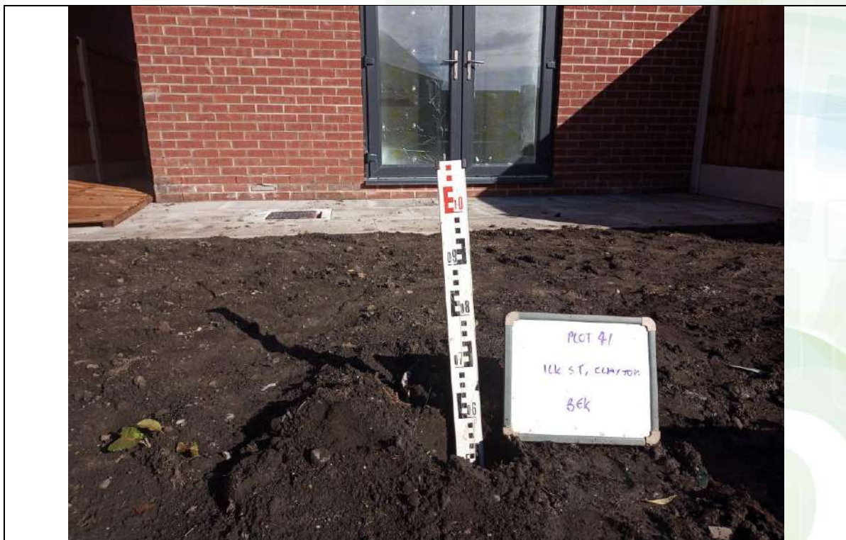
Photograph 2: Validation of Garden Capping Thickness
