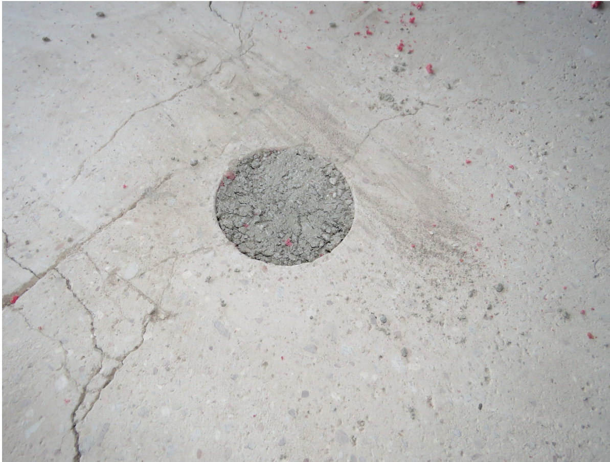
02-08 Close up view of one of the intrusive investigation cores to the floor slab, now backfilled with concrete.
