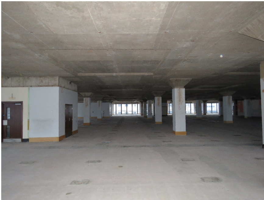
02-05 Looking west across the podium.
