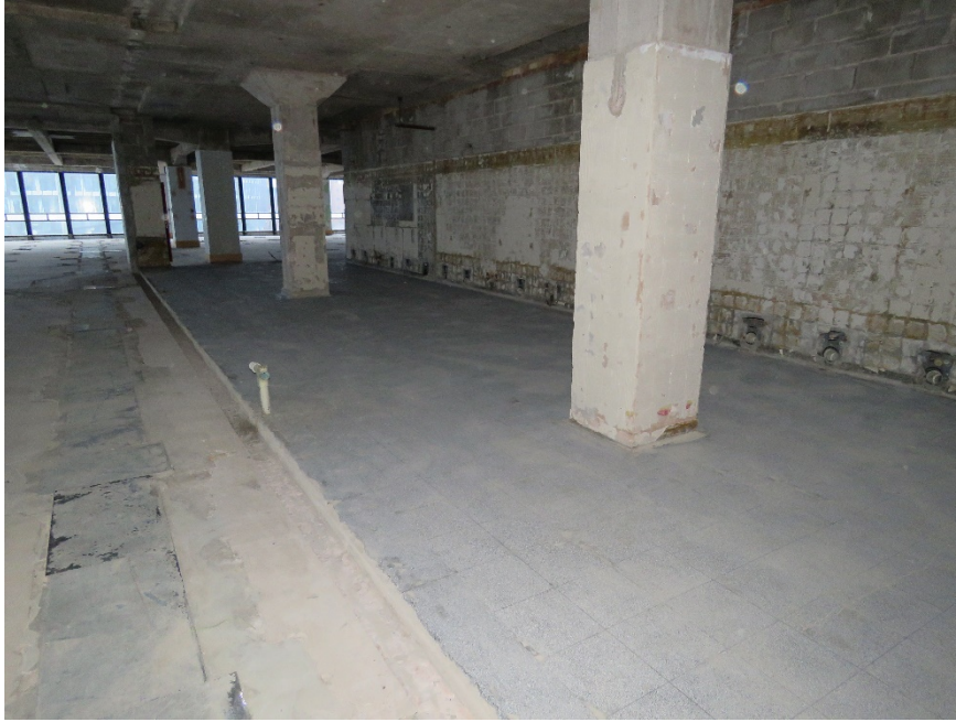
02-10 View north showing the extent of surviving terrazzo tiles to the WC area.
