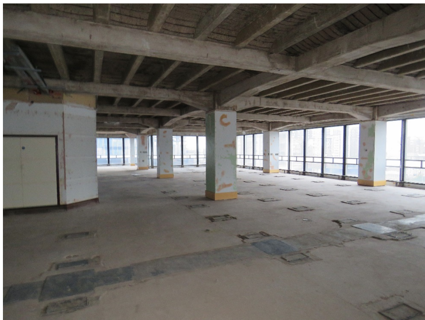
02-01 Looking northwest into the office-tower.
