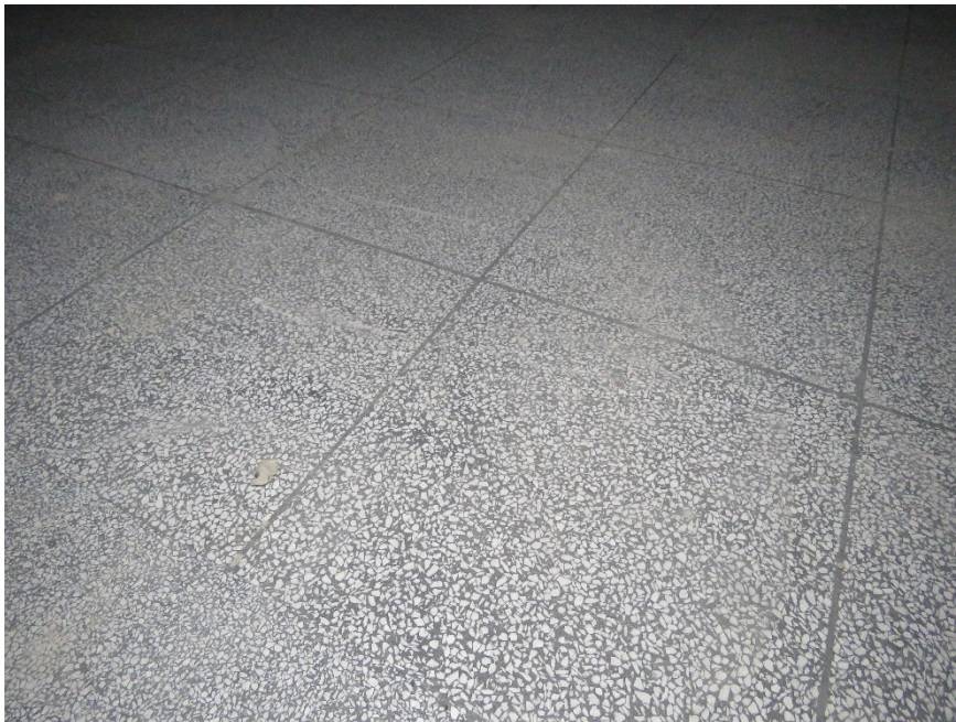
02-11 Close up view of the uncovered terrazzo tiles.
