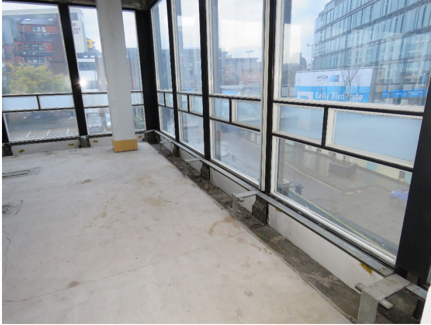
02-06 View of the floorplates perimeter following the strip out of the Weathermaster system. Note the steel frame of the boxing in is connected back to the buildings structure and curtain walling.
