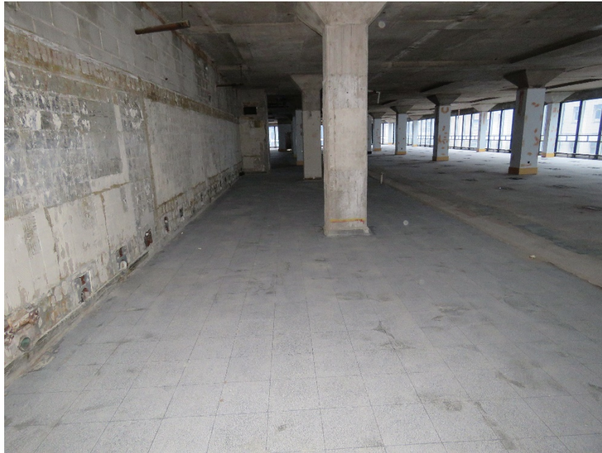
02-12 View south over the area of uncovered terrazzo tiles.
