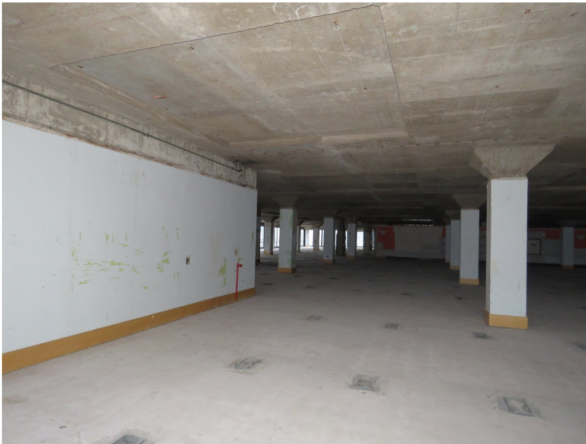
02-07 Looking north across the podium.
