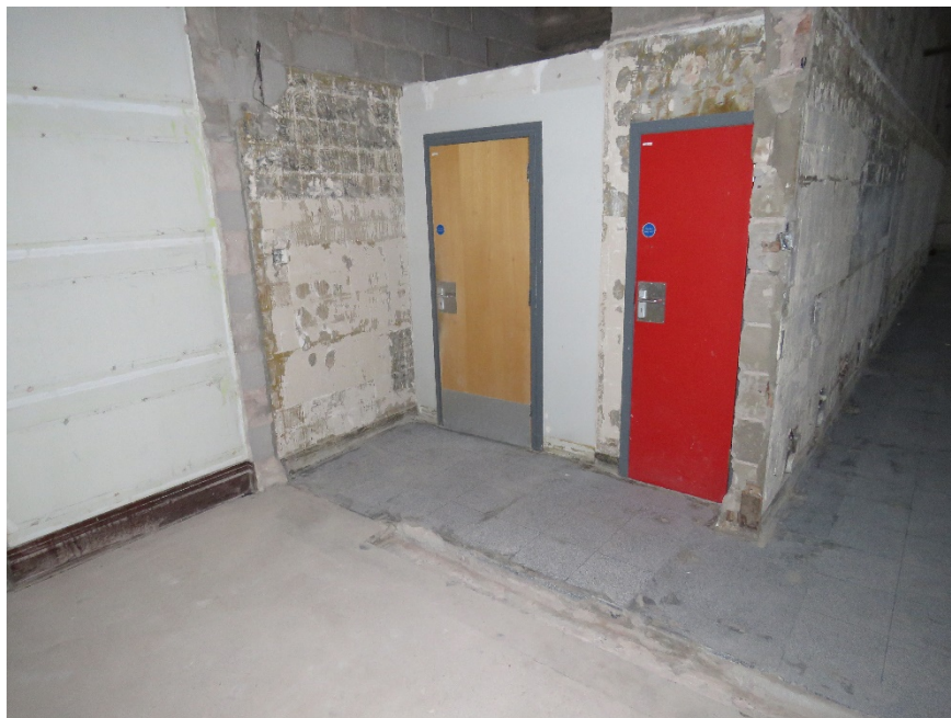
02-13 The tiling continues into the storage cupboards.
