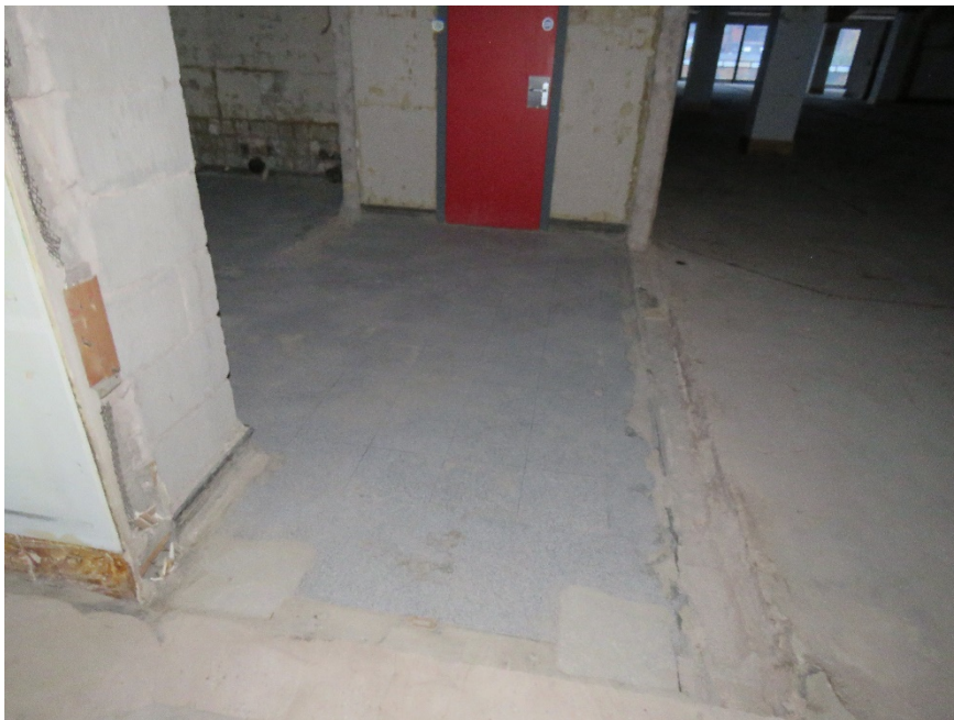
02-09 View of the terrazzo tiles within the location of the WC's to the west of the lift core.
