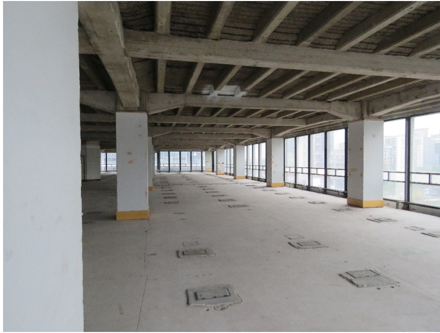
02-02 Looking west into the office-tower.
