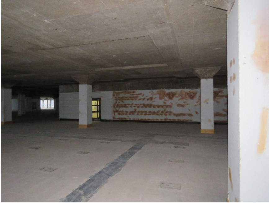
02-04 Looking west towards the stair, escalator and lift core.
