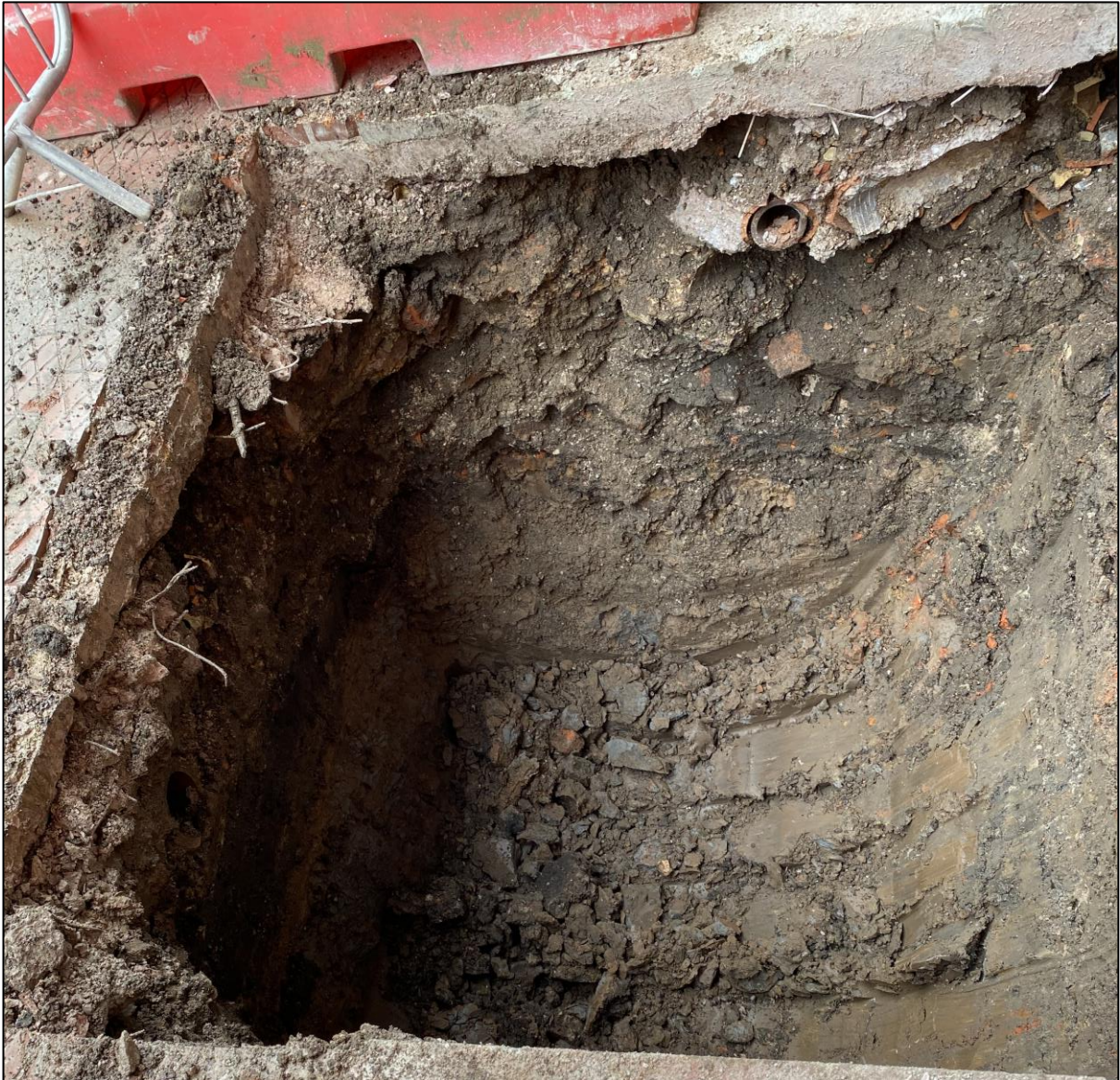
Plate 2: Natural clay within trial pit along southern interior wall
