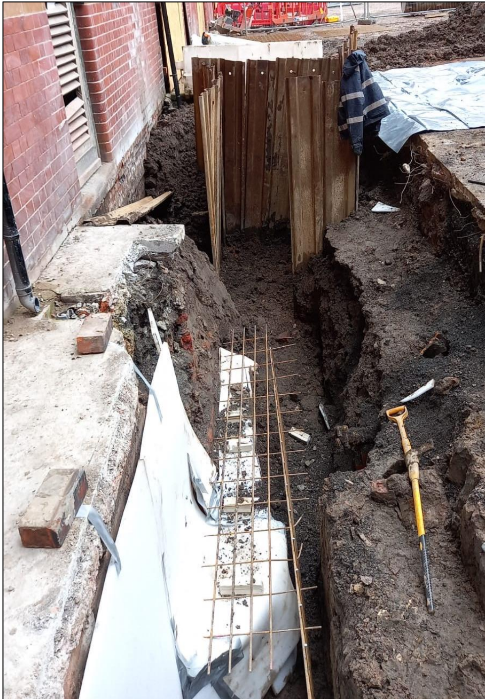
Plate 1: Trial pit along northern interior wall
