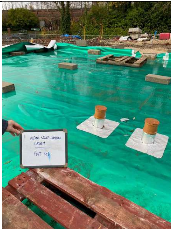
Photograph 5: Validation of Gas Membrane Installation
