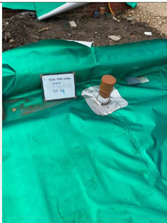
Photograph 6: Validation of Gas Membrane Installation
