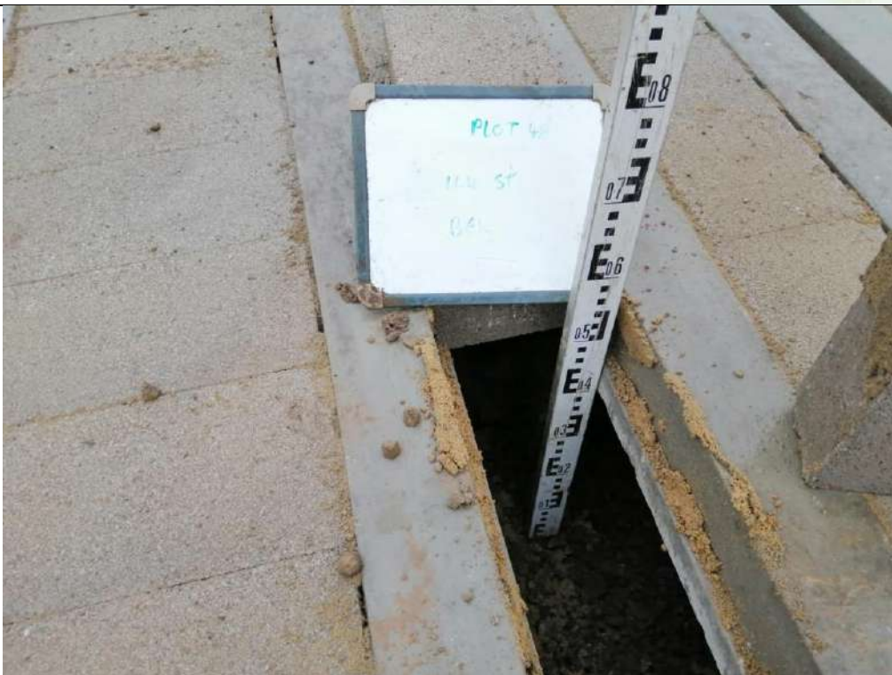
Photograph 4: Validation of Sub-Floor Void Space (min 150 mm)
