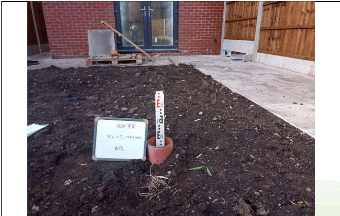
Photograph 1: Validation of Garden Capping Thickness
