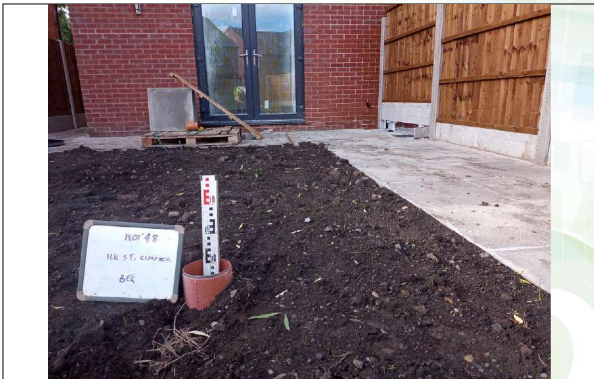
Photograph 2: Validation of Garden Capping Thickness
