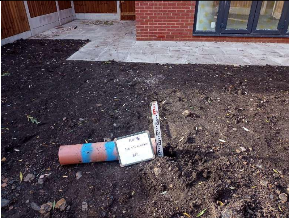
Photograph 1: Validation of Garden Capping Thickness
