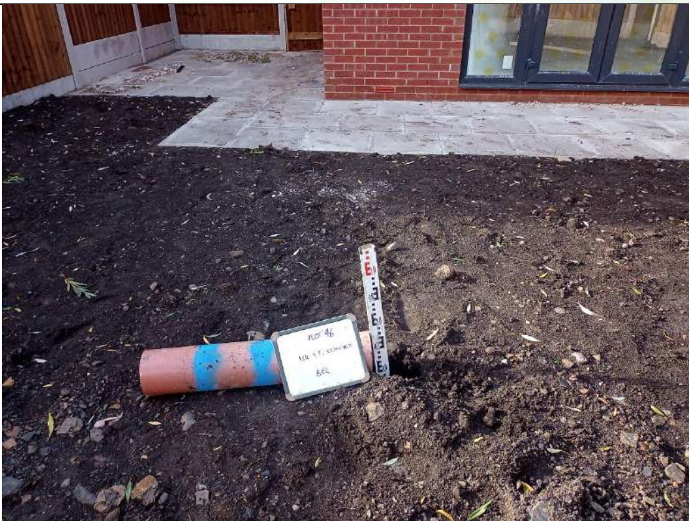
Photograph 2: Validation of Garden Capping Thickness
