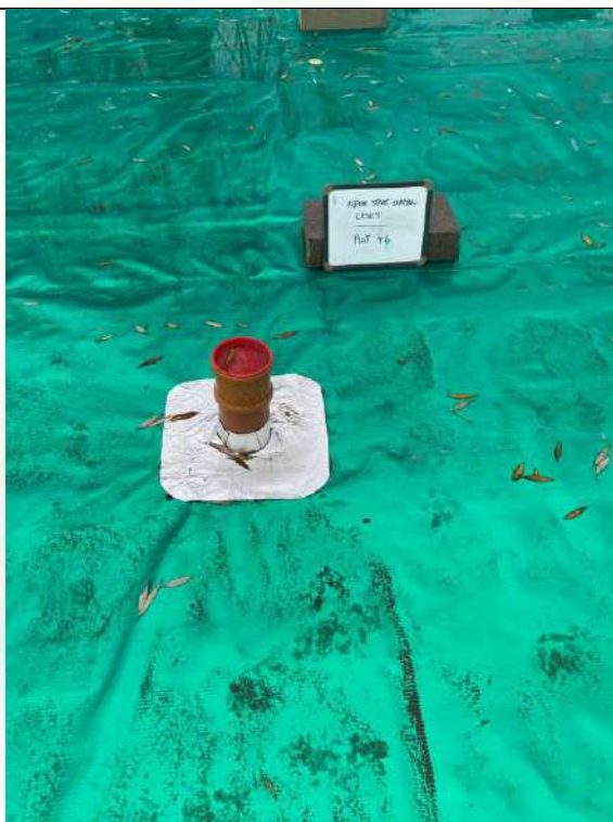
Photograph 6: Validation of Gas Membrane Installation
