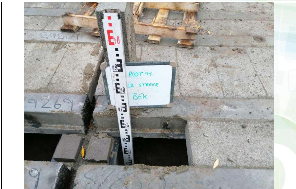
Photograph 4: Validation of Sub-Floor Void Space (min 150 mm)
