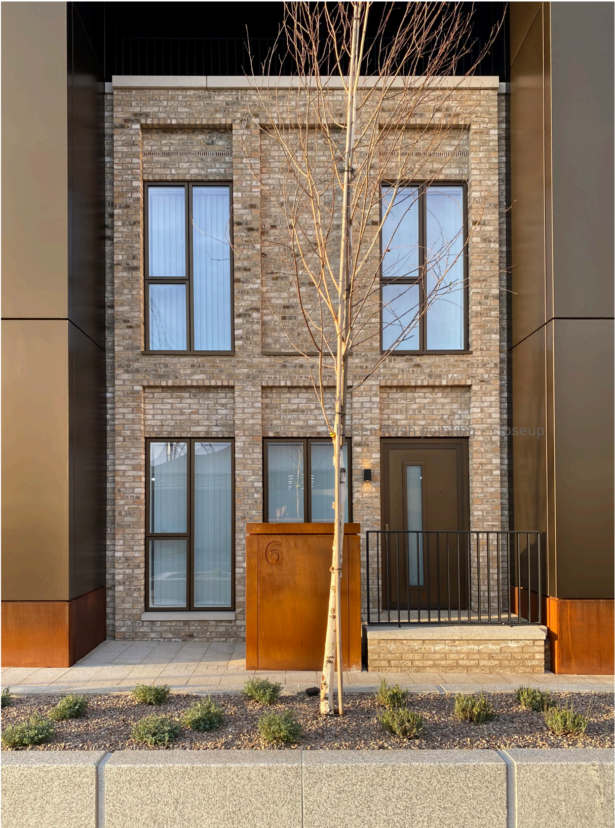
Crown Street Phase 1 - Completed brickwork Indicative brickwork, mortar and pointing only Photographed 06.11.20
