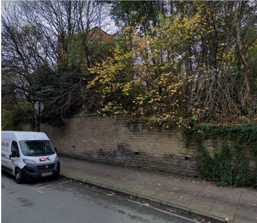
Figure 17: Site photo. Late-20 th century stone boundary wall and mature vegetation.
