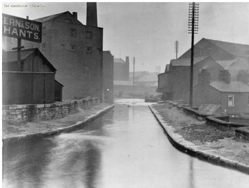
Figure 9: 1906 Photograph looking east across the aqueduct – this photo illustrates the industrial character of the area in the early 20 th century with industrial buildings hard-up against the edge of the canal. Note the range and variety of building heights and forms.
