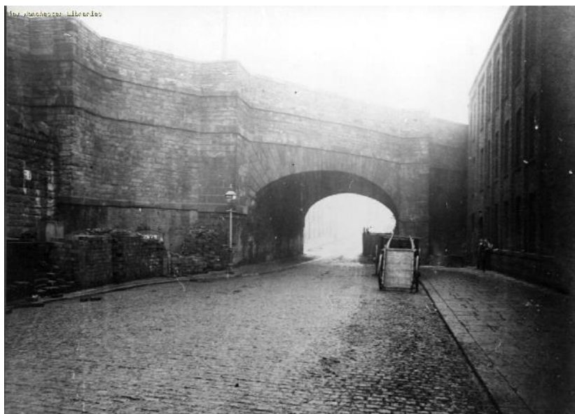
Figure 7: 1896 Photograph of south west side of Aqueduct – this early photograph illustrates the north façade of the Packing Case Manufactory works which historically occupied the Site (right side of image) and illustrates that buildings were built hard-up alongside the aqueduct, canal, and to the back of pavement line. The late-19 th century photo of the aqueduct looking south along Store Street allows for its architectural expression to be fully appreciated.
