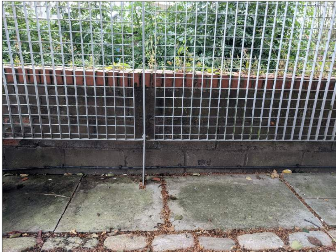
Plate 4: Detail of above showing modern construction
