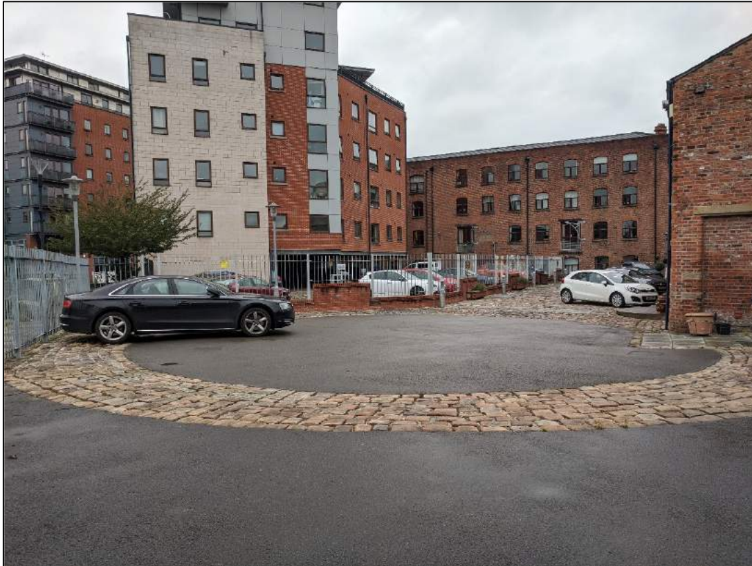
Plate 1: General shot of site showing Junction Lead Mills in the background
