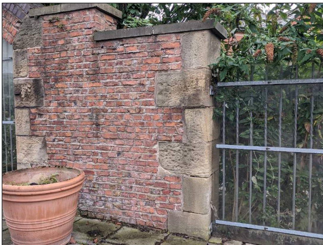
Plate 15: Sandstone quoins to west end
