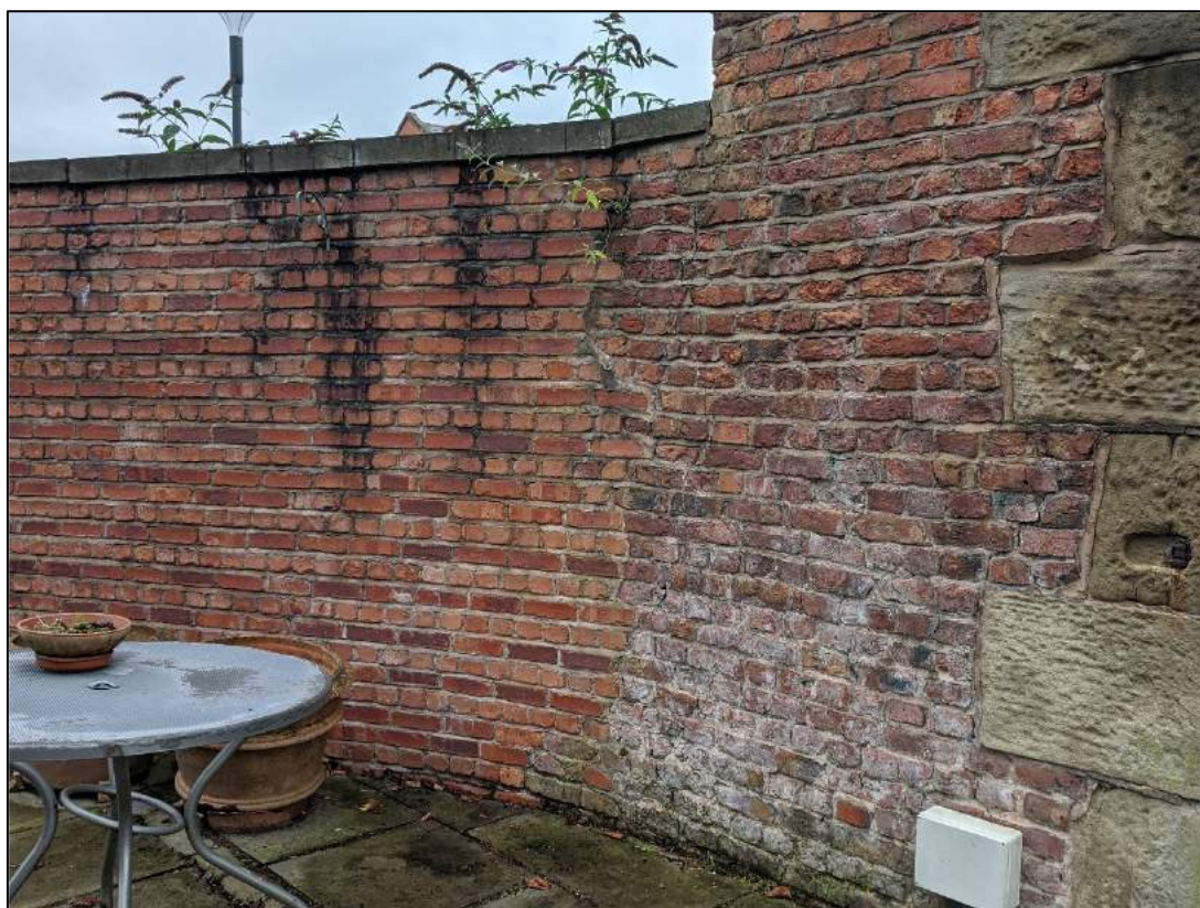
Plate 13: Detail of joint between original wall and rebuild
