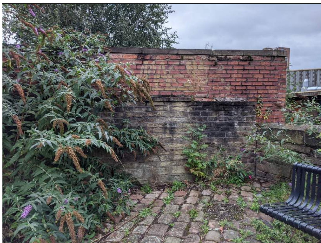
Plate 16: East end of wall from canal tow path showing brick over stone
