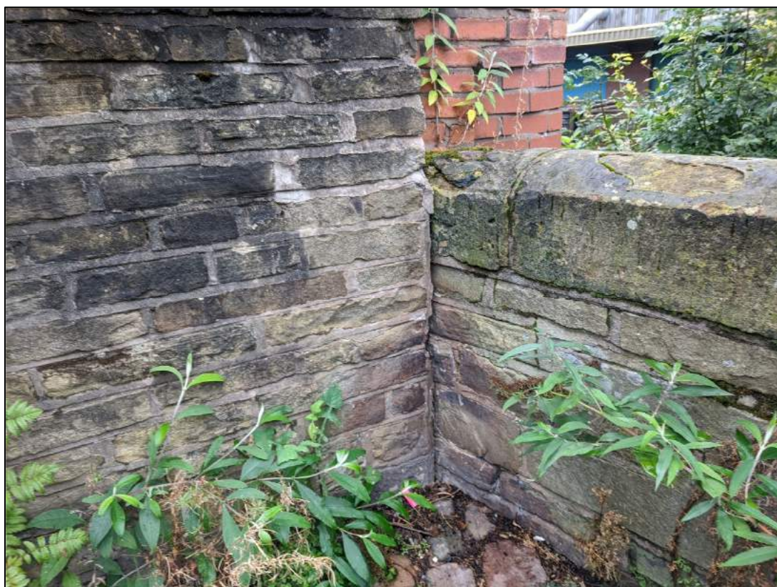
Plate 17: Stone boundary wall shown above butting up to canal wall (right)
