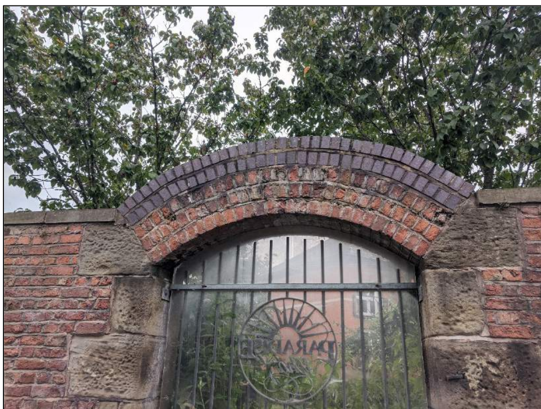
Plate 14: Detail showing rebuilt lintel
