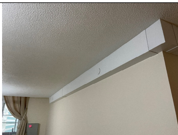
Living Area (being used as an office)
