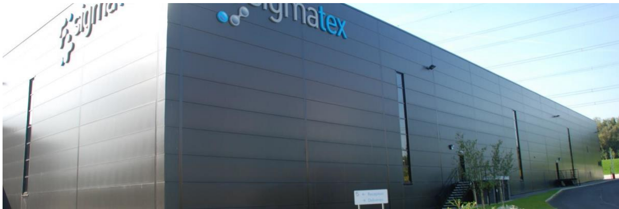
An example of black "Colorcoat Prisma" cladding
