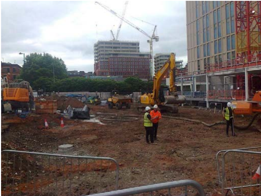
Photo 1: Infilled basement and piling mat – piling operations being undertaken
