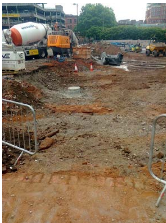
Photo 2: Imported materials used to infill basement and construct piling mat
