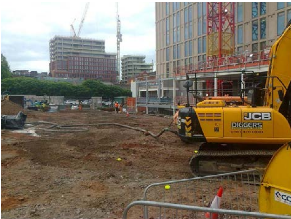
Photo 4: Infilled basement and piling mat – piling operations being undertaken
