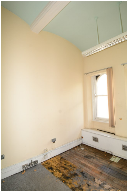
Existing partition wall between rooms 04-003 & 04-003a
