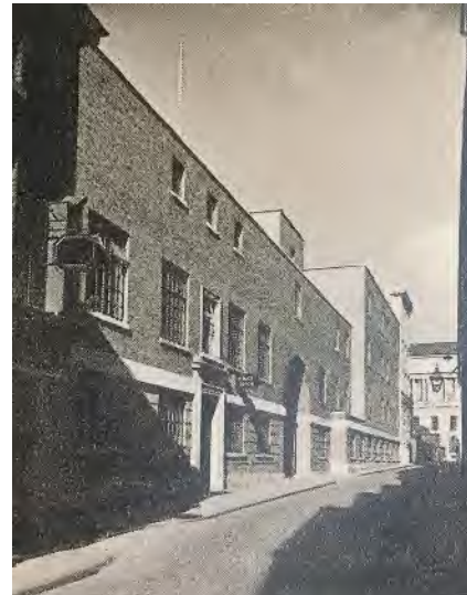
1937 - View east along Bootle Street
