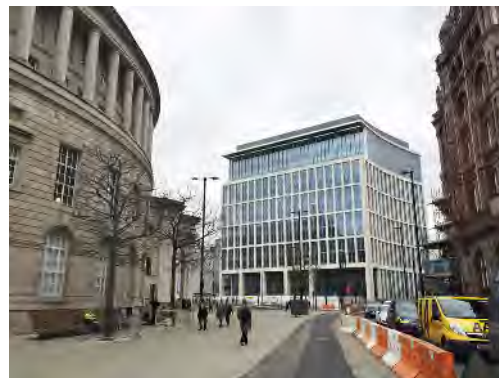
New office development to the east of the square
