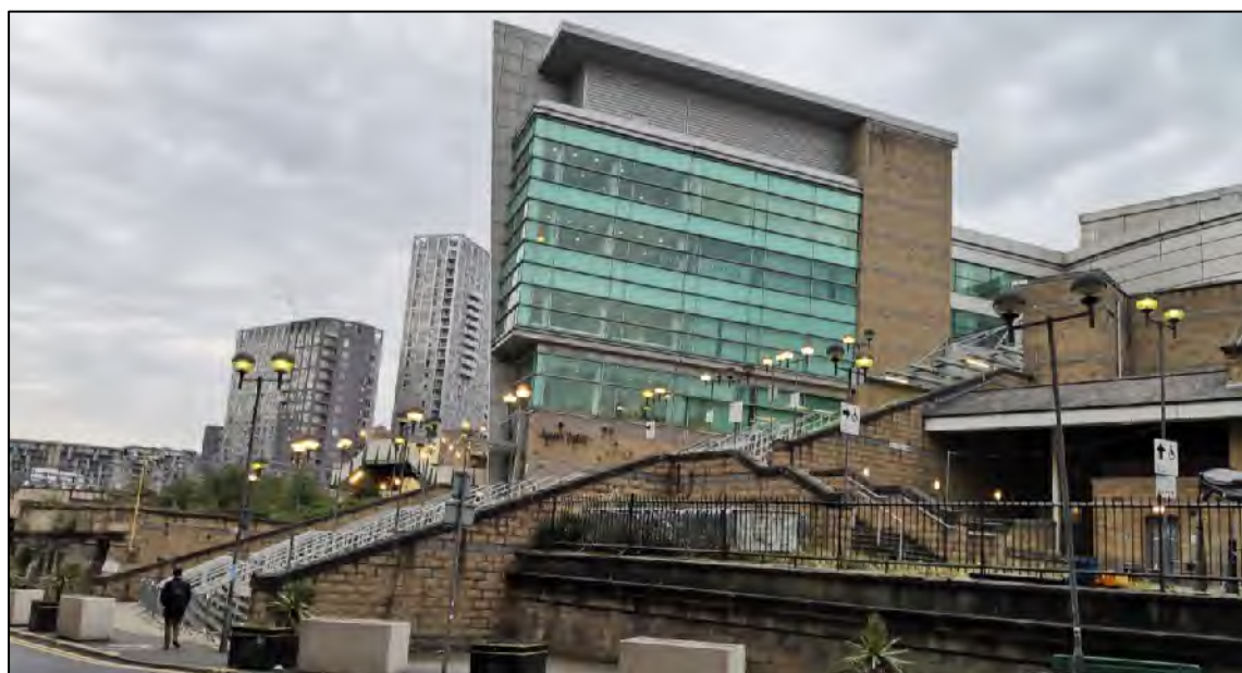
Plate 41: View of Manchester AO Arena, with mid- and high-rise buildings in the Manchester skyline, looking west
