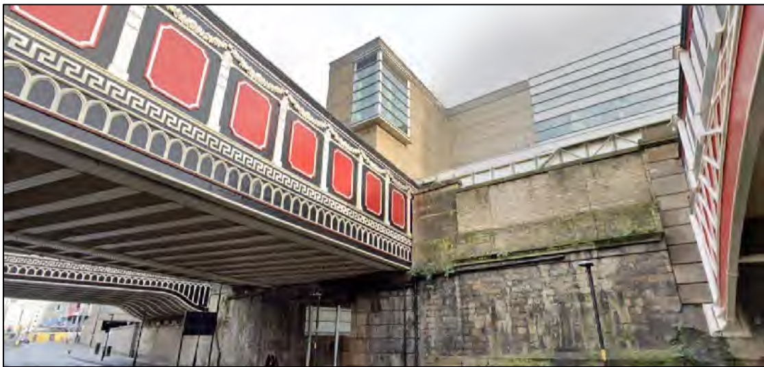
Plate 35: Middle Bridge, looking east
