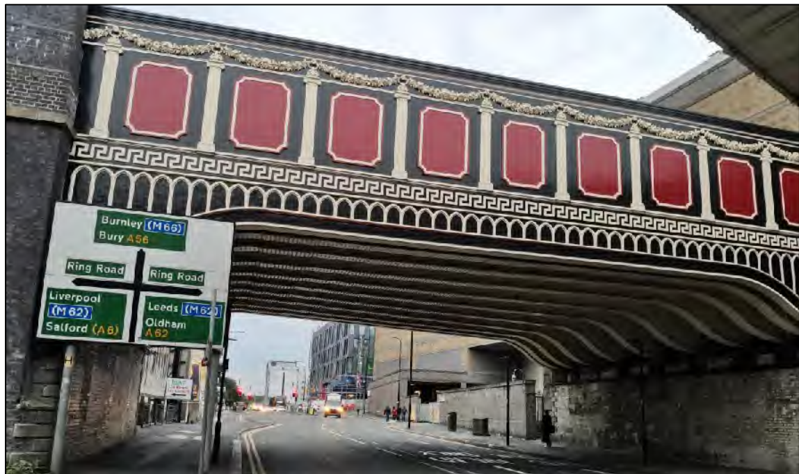
Plate 29: North Bridge, looking north-west
