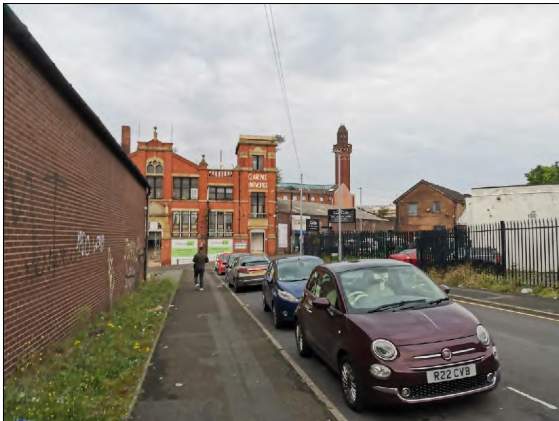
Plate 45: Viewpoint of the former Clarence Hat Works building, looking north-west
