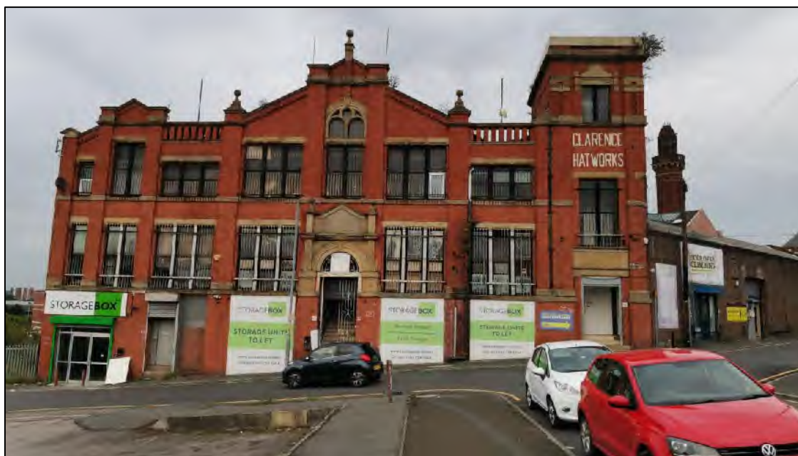
Plate 26: Former Clarence Hat Works Building, looking north-west from Dutton Street
