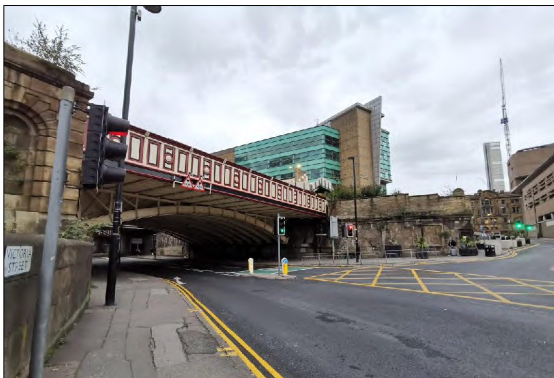
Plate 39: View of Stephenson Bridge from Victoria Street and Victoria Station to the right, looking east
