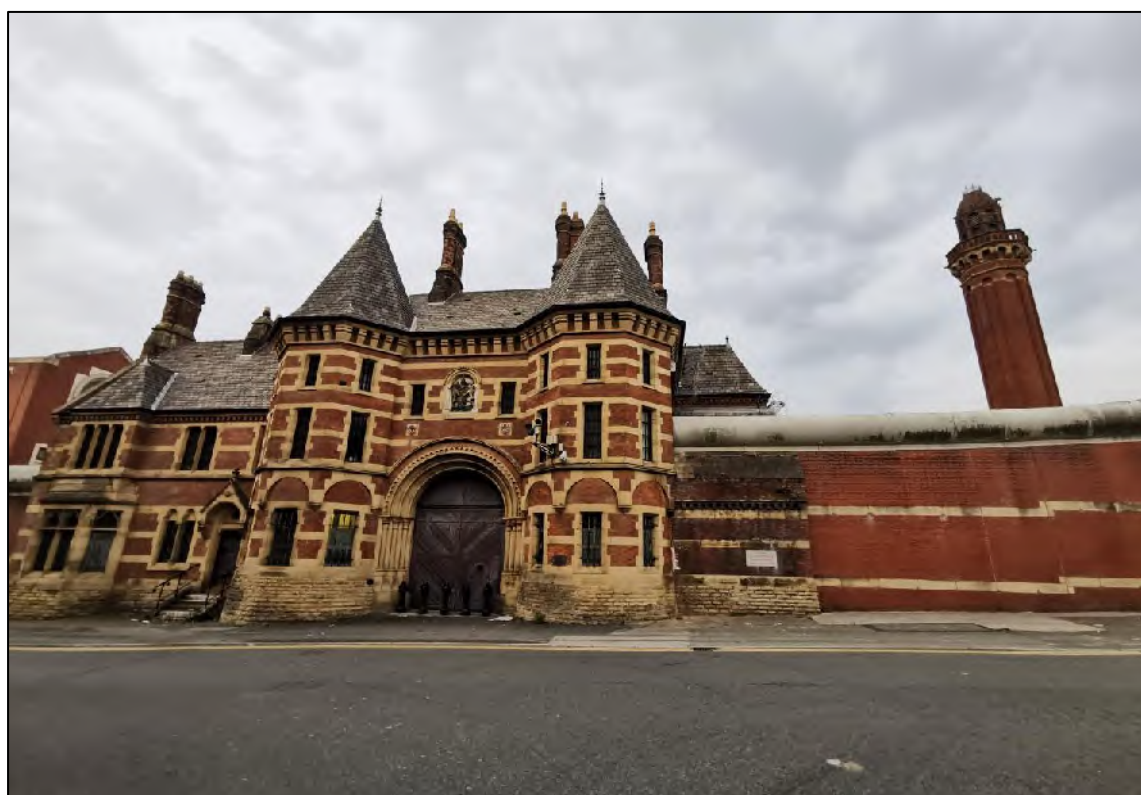
Plate 28: Southern façade of the HMP Manchester Gatehouse, and Strangeways tower. Image taken facing the north-west, looking away from the site.
