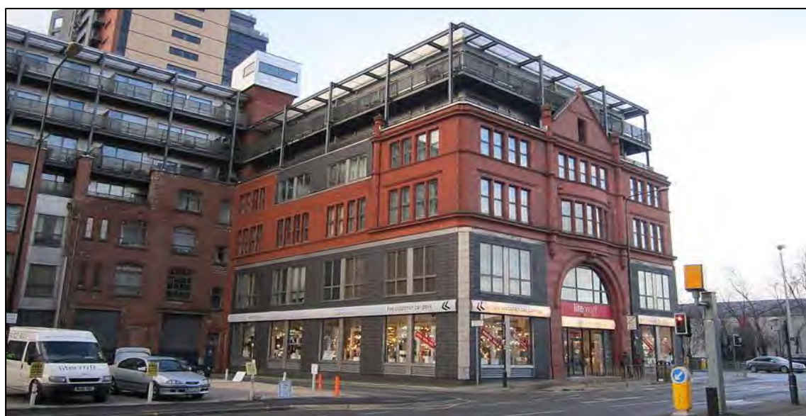
Plate 27: Former Motor Works building, regenerated into commercial and residential units
