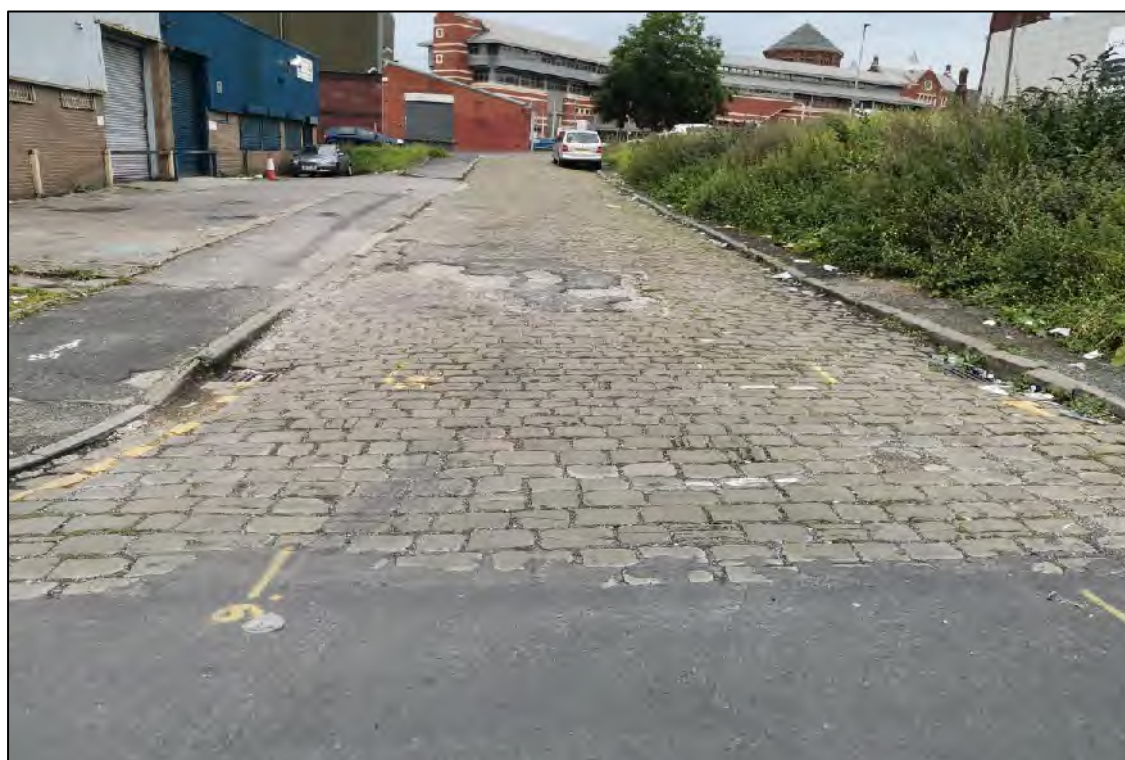
Plate 24: Cobbled surface of Newcombe Street, to the north-west of the Site
