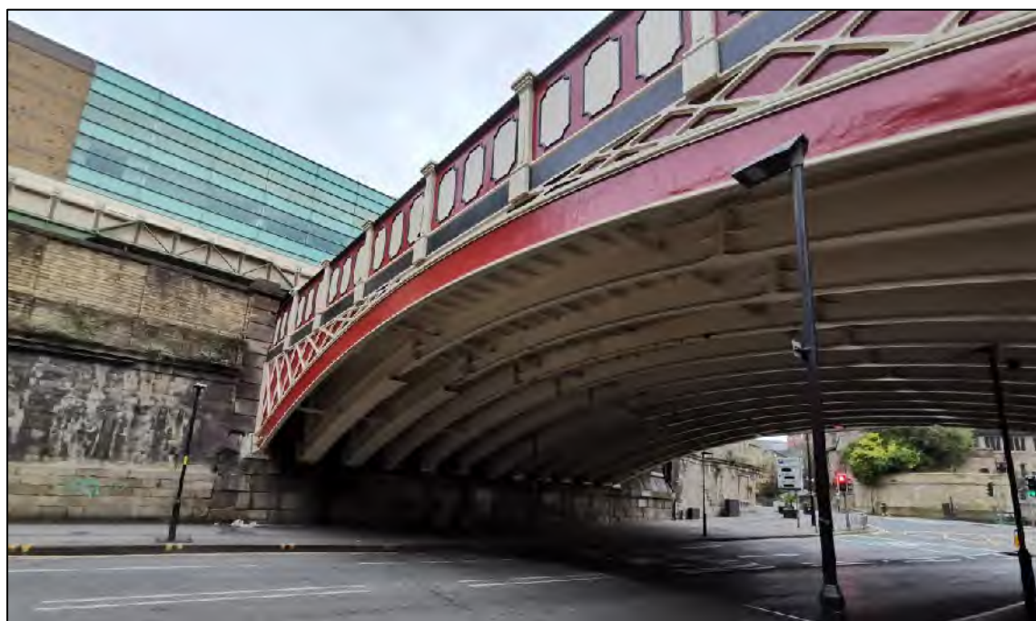
Plate 34: Stephenson Bridge, looking south-east
