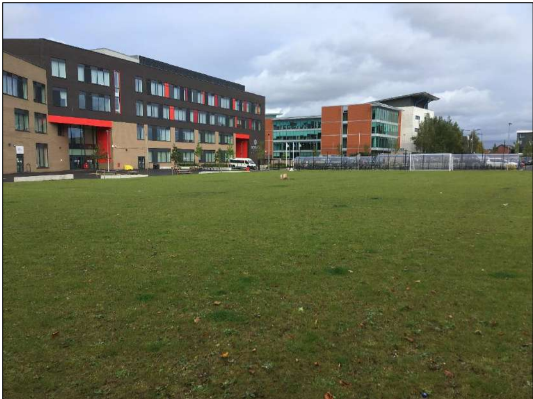
Figure 1-2 At southeast of pitch looking towards the northwest
