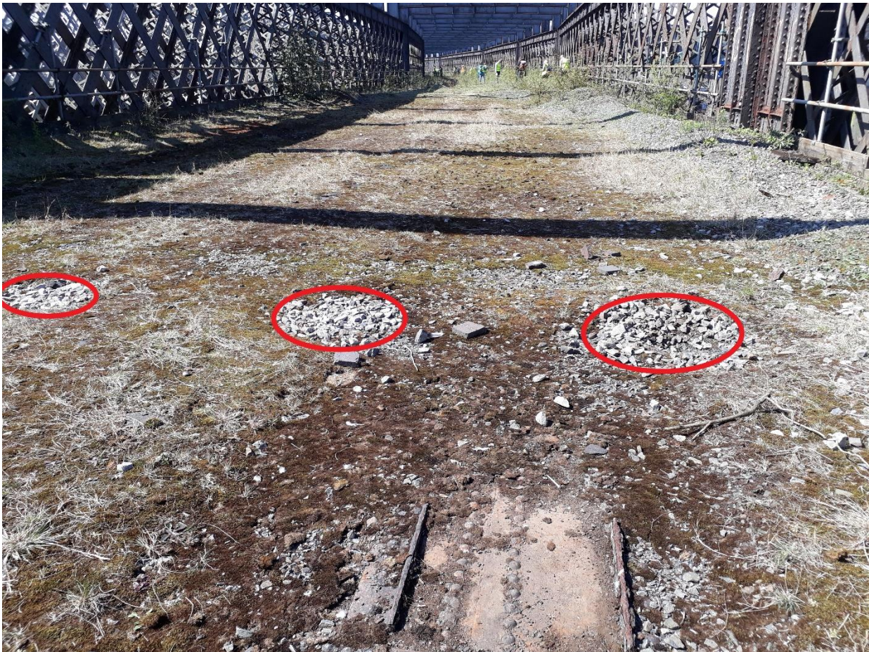
Figure 3-1: Location of Drainage Inlets at Viaduct Deck Level
