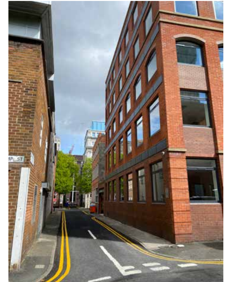
Figure 4.3 The west elevation of the Site, as viewed from Camp Street, looking north
