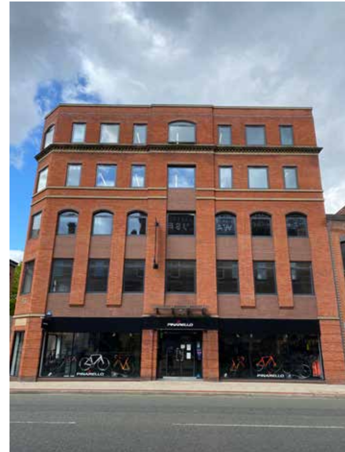
Figure 4.2 The principal south elevation of the Site is regularly fenestrated and divided into a 3-1-3 bay pattern
