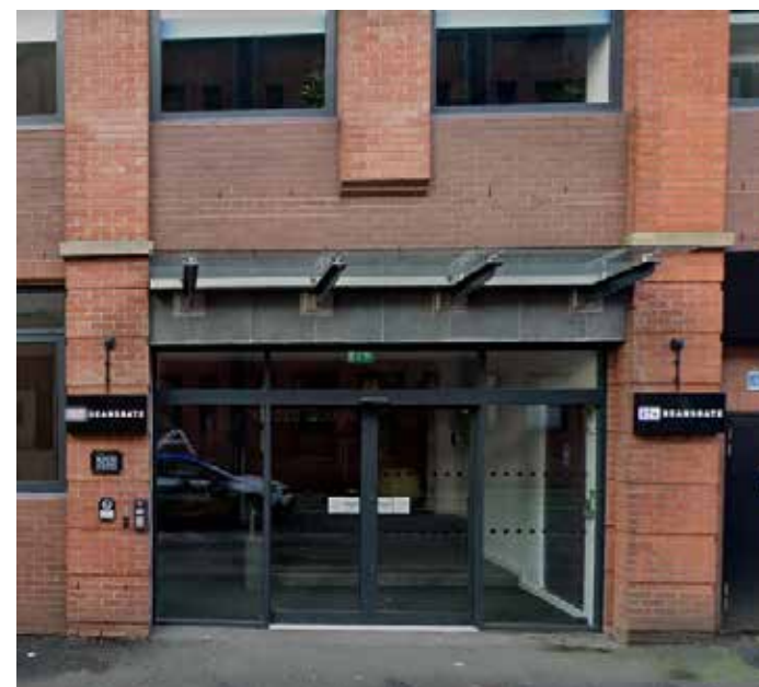
Figure 6.4 Existing main entrance located on the west elevation, fronting Camp Street Drawing produced by Calderpeel Architects
