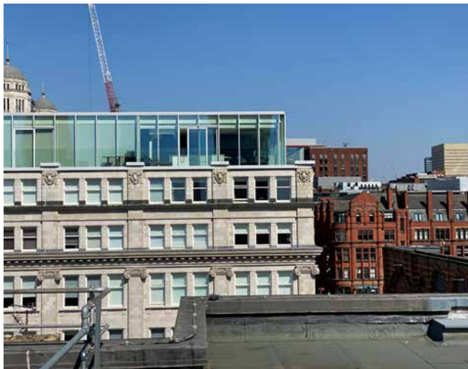
Figure 4.5 Views of tall buildings located further east along Deansgate, as seen from the roof of the Site. In particular, no. 2 John Street, with its historic stone facade, capped with a contemporary glass upward extension, is highly visible.
