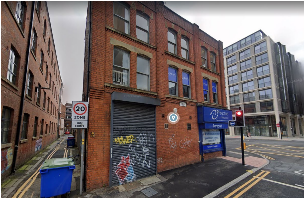
Photograph 5: Existing side elevation
