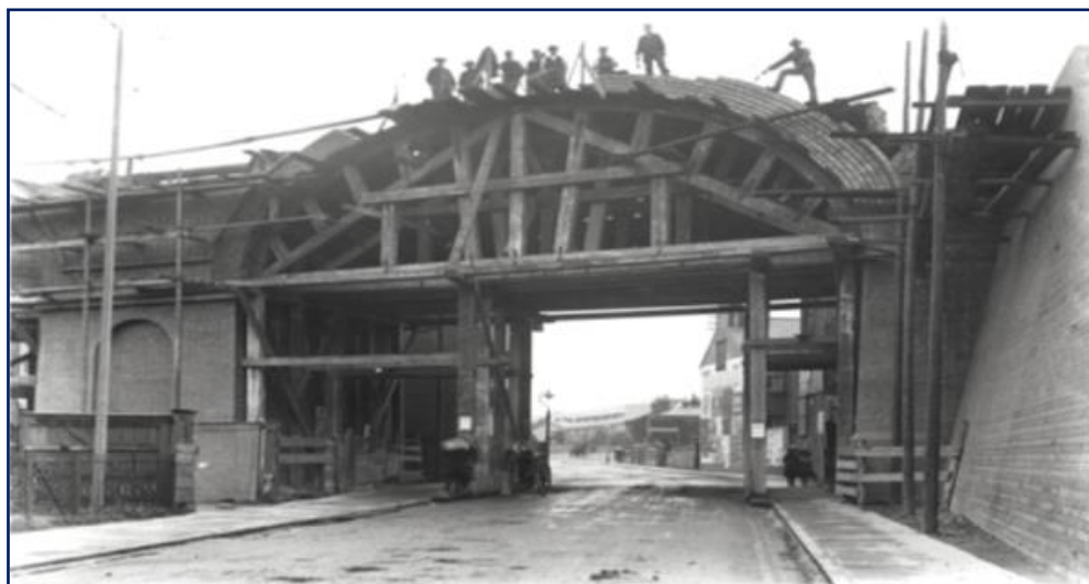
Image 3: Source: Workers constructing railway viaduct, 1903 National Transportation Archive.
