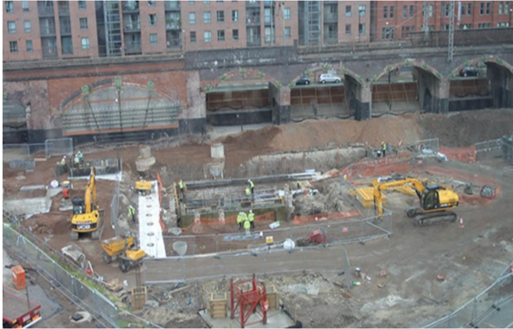
Image 1: The ground works for the construction of the Manchester HOME development in 2013. The three Arches are shown directly to the north of the construction site. Image source: www.homemcr.org )
