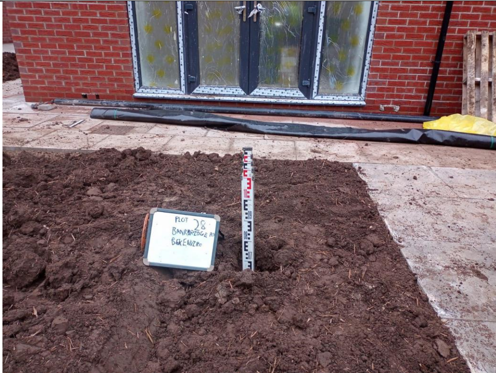
Photograph 1: Validation of Garden Capping Thickness
