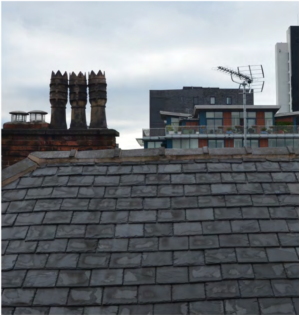
existing slates to neighbouring 56 Dale Street
