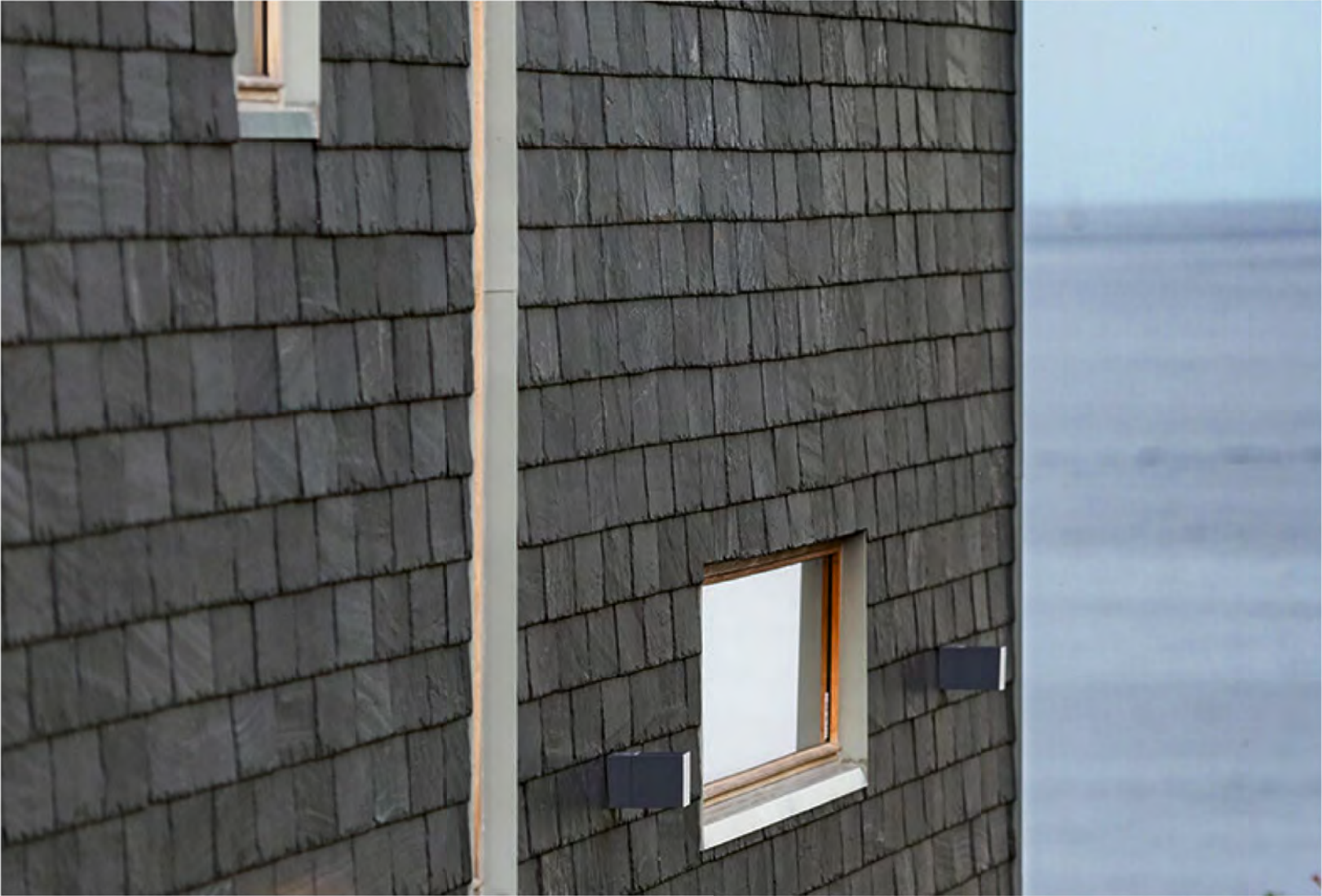
proposed Cupaclad natural rainscreen cladding
