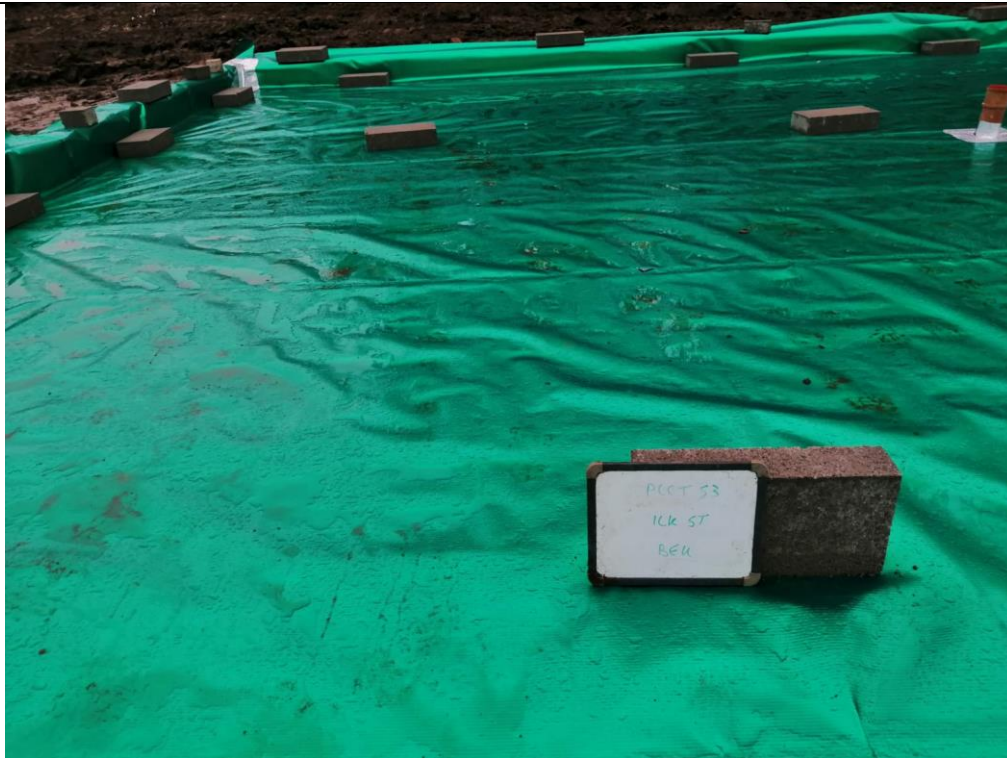
Photograph 7: Validation of Gas Membrane Installation
