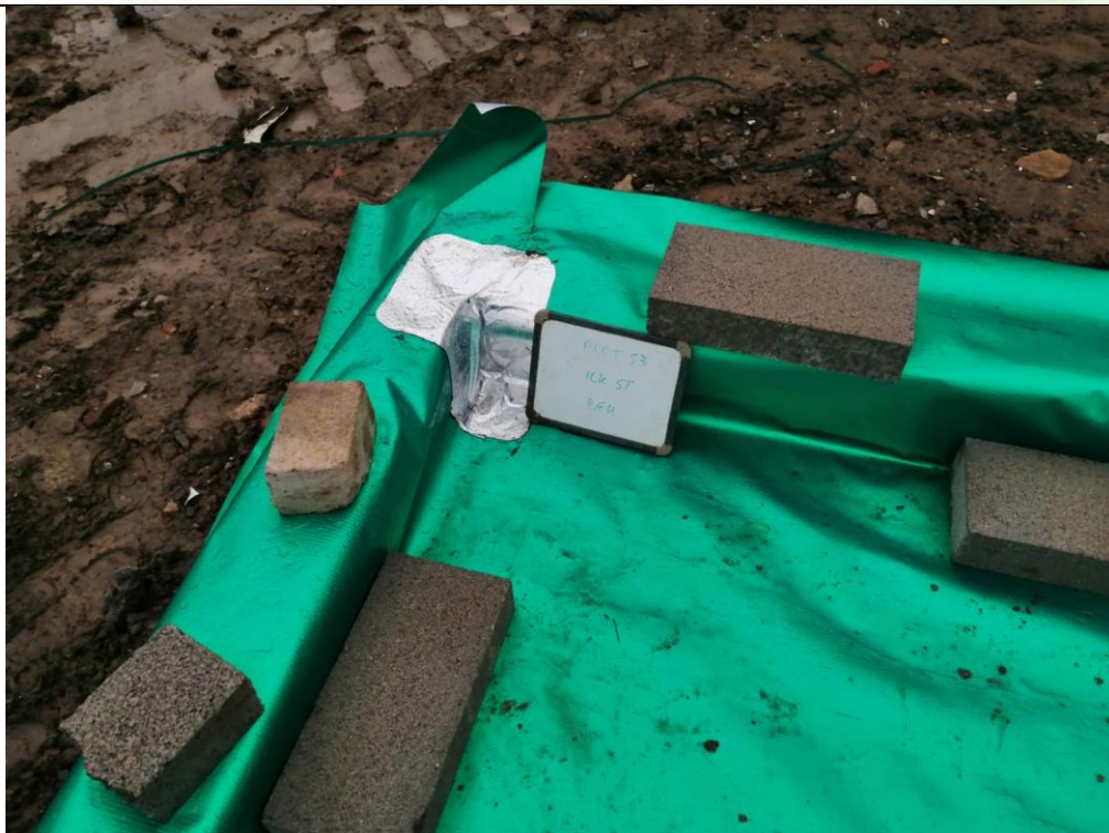
Photograph 6: Validation of Gas Membrane Installation
