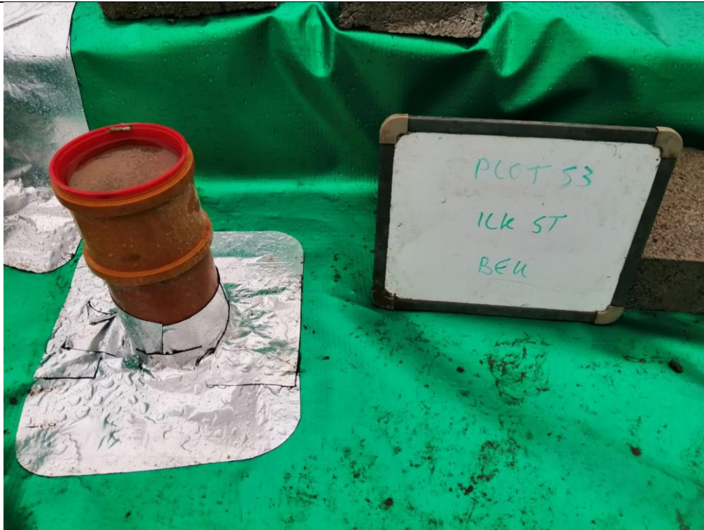
Photograph 5: Validation of Gas Membrane Installation
