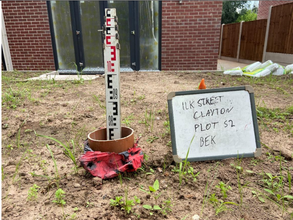
Photograph 1: Validation of Garden Capping Thickness (Plot 53, not 52)
