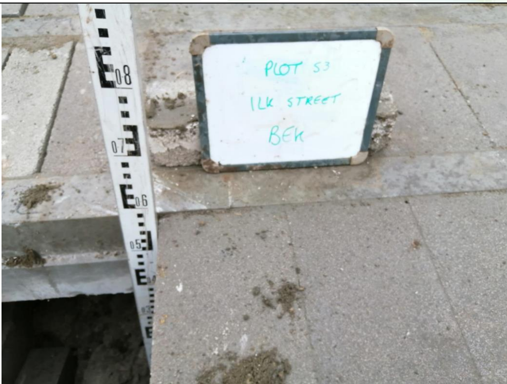
Photograph 4: Validation of Sub-Floor Void Space (min 150 mm)
