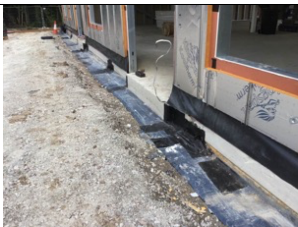
Perimeter edge and stanchions sealed
