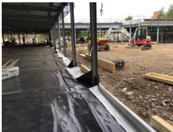
SAGM being pick tested around a stanchion
