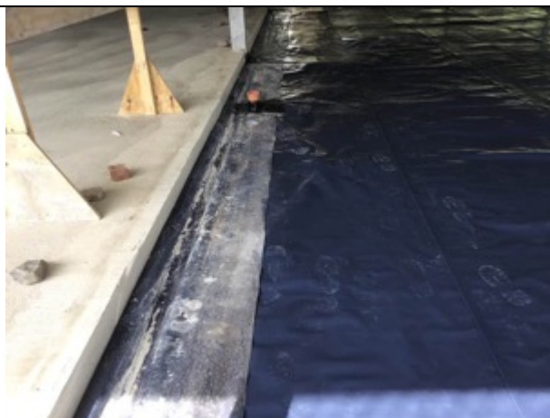
Joint to previously installed membrane
