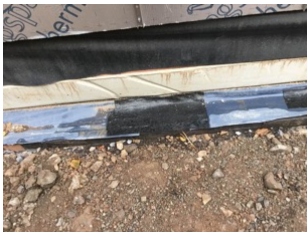
Patch repairs
