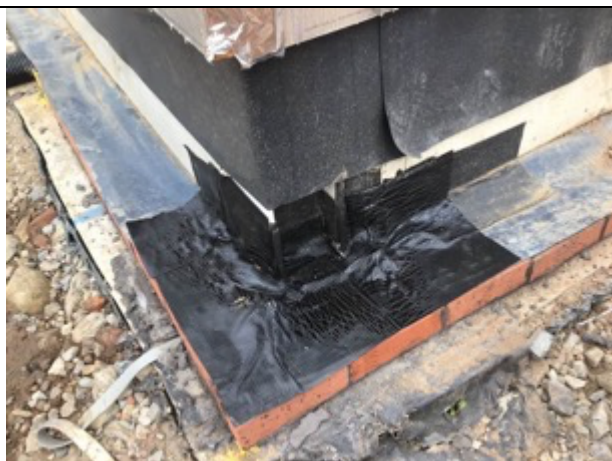
Perimeter corner repair
