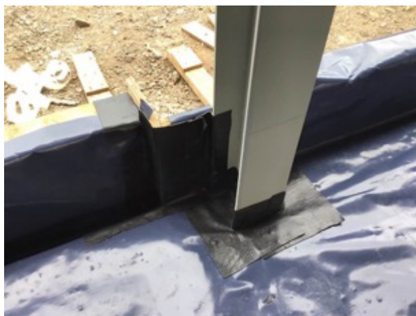
Sealed pipe penetration
