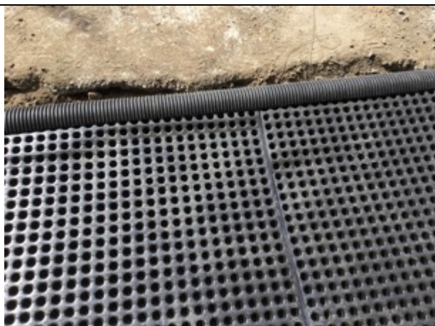
Vent mat inserted into slotted collection pipe
