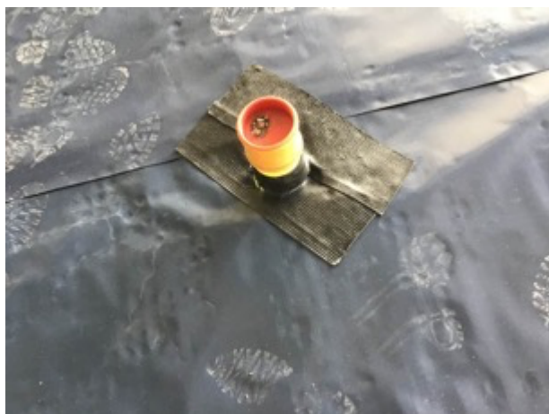
Stanchion seal using SAGM
