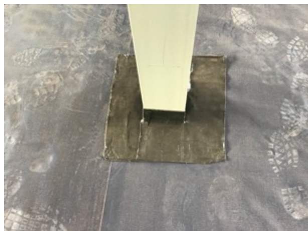
Pipe seal using SAGM
