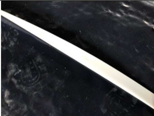
Sealed double sided butyl tape membrane joint
