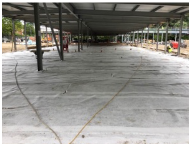
Vent mat connected to perimeter T piece
