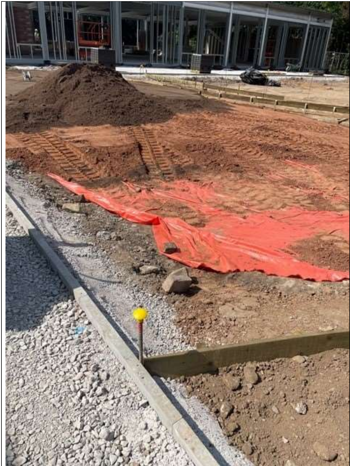
Plate 2: View showing the installation of the geotextile membrane beneath the landscaped areas.
