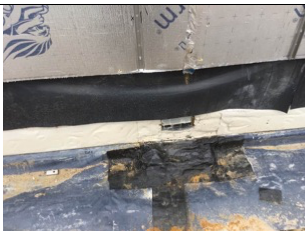
Stanchion seal using SAGM
