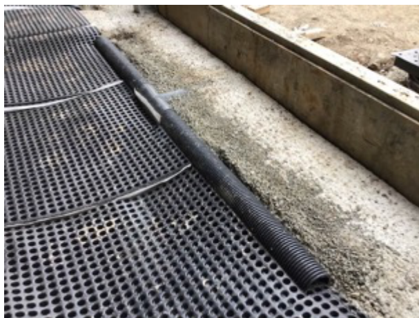
Vent mat joining to perimeter T piece
