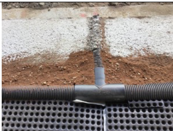
"T" piece with slotted pipe
