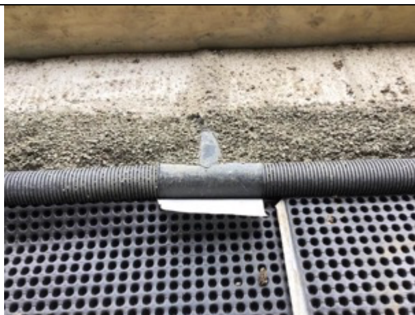
Vent mat joining to perimeter T piece
