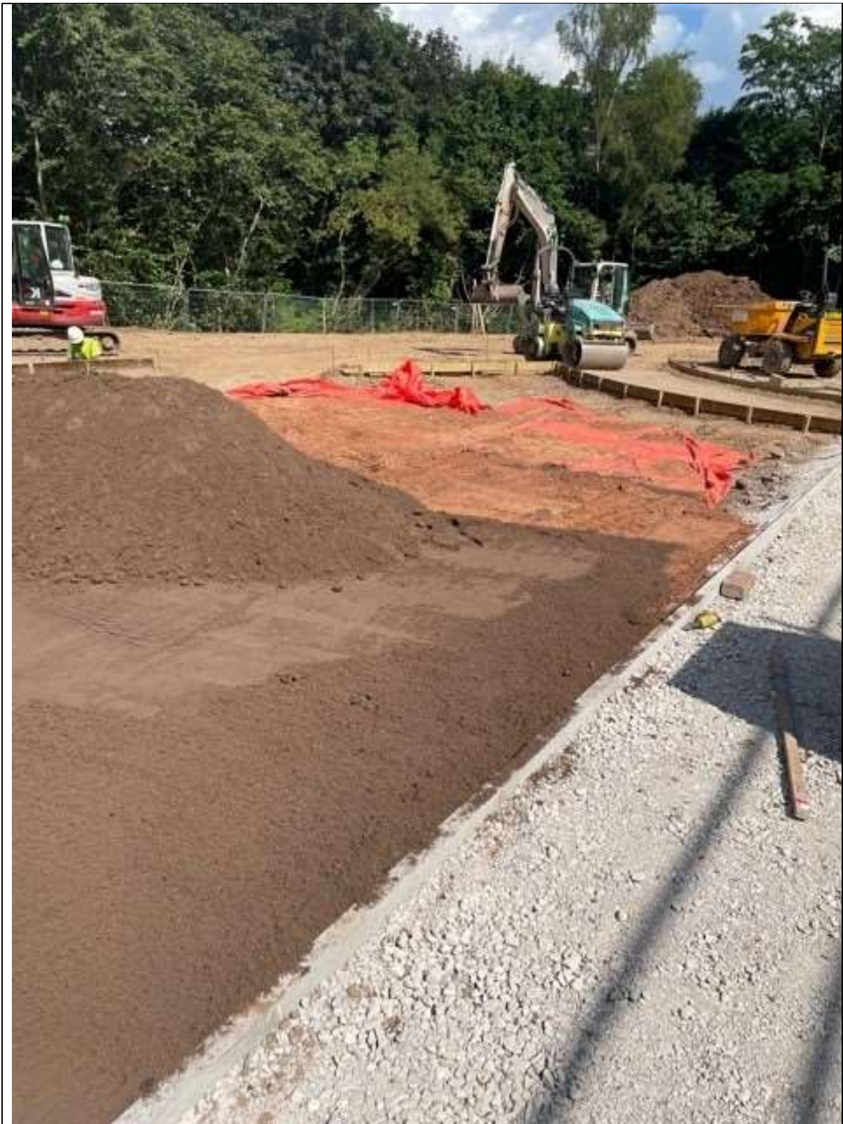
Plate 3: View showing the installation of the geotextile membrane beneath the landscaped areas.
