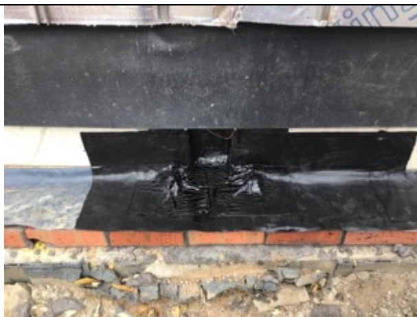
Perimeter steel repair
