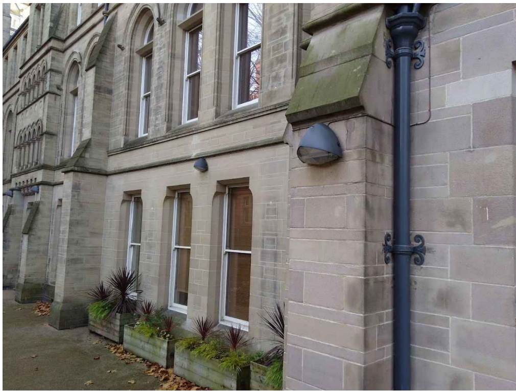
Example of existing light fitting on building
