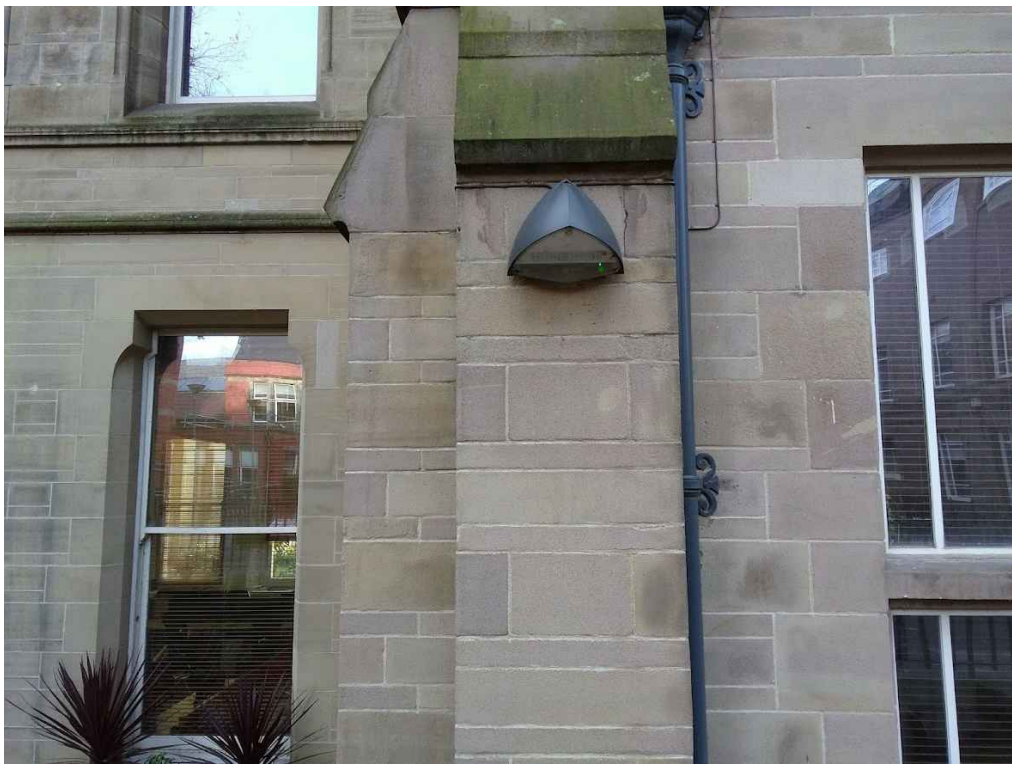
Example of existing light fitting on building
