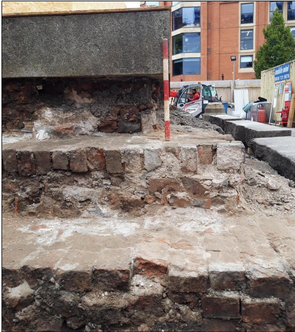
Plate 3: Tiered brick base – east side, looking west
