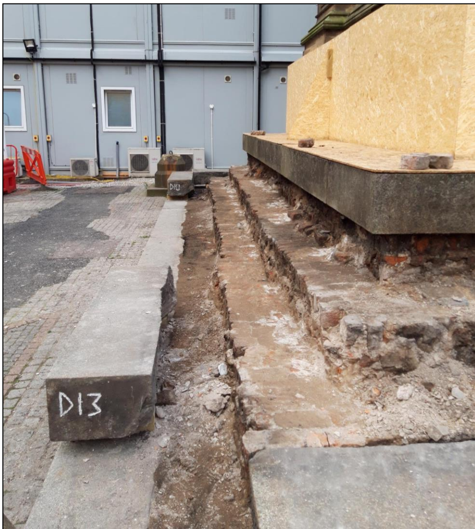
Plate 2: Brick base below the marble stepped base and statue – west side looking north
