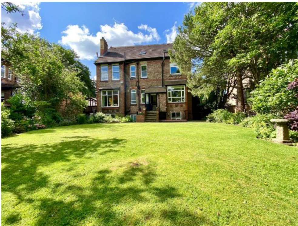
Rear of 25 Parkfield Road South
