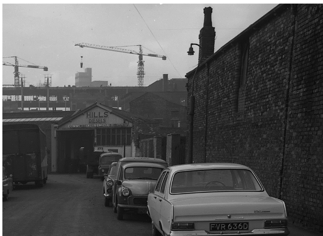
Figure 16 – Looking north-west along Tariff Street towards the Site (behind the wall to the right) in 1966, showing the entrance into the rear of the Site.
