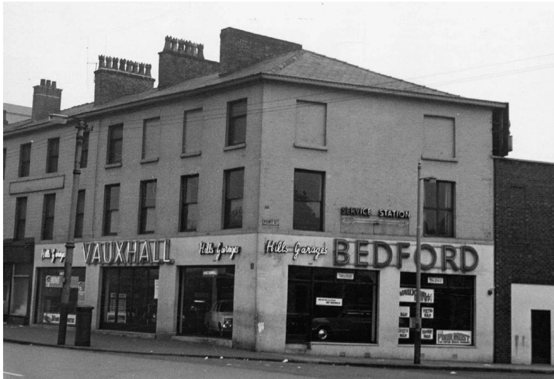
Figure 17 – A view of the north corner of the Site in 1967, showing the original early-19 th century buildings on the corner of Port Street (right) and Great Ancoats Street (left).
