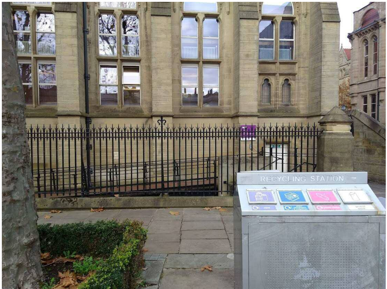
Fig 3: John Owens South Elevation from Burlington Street
