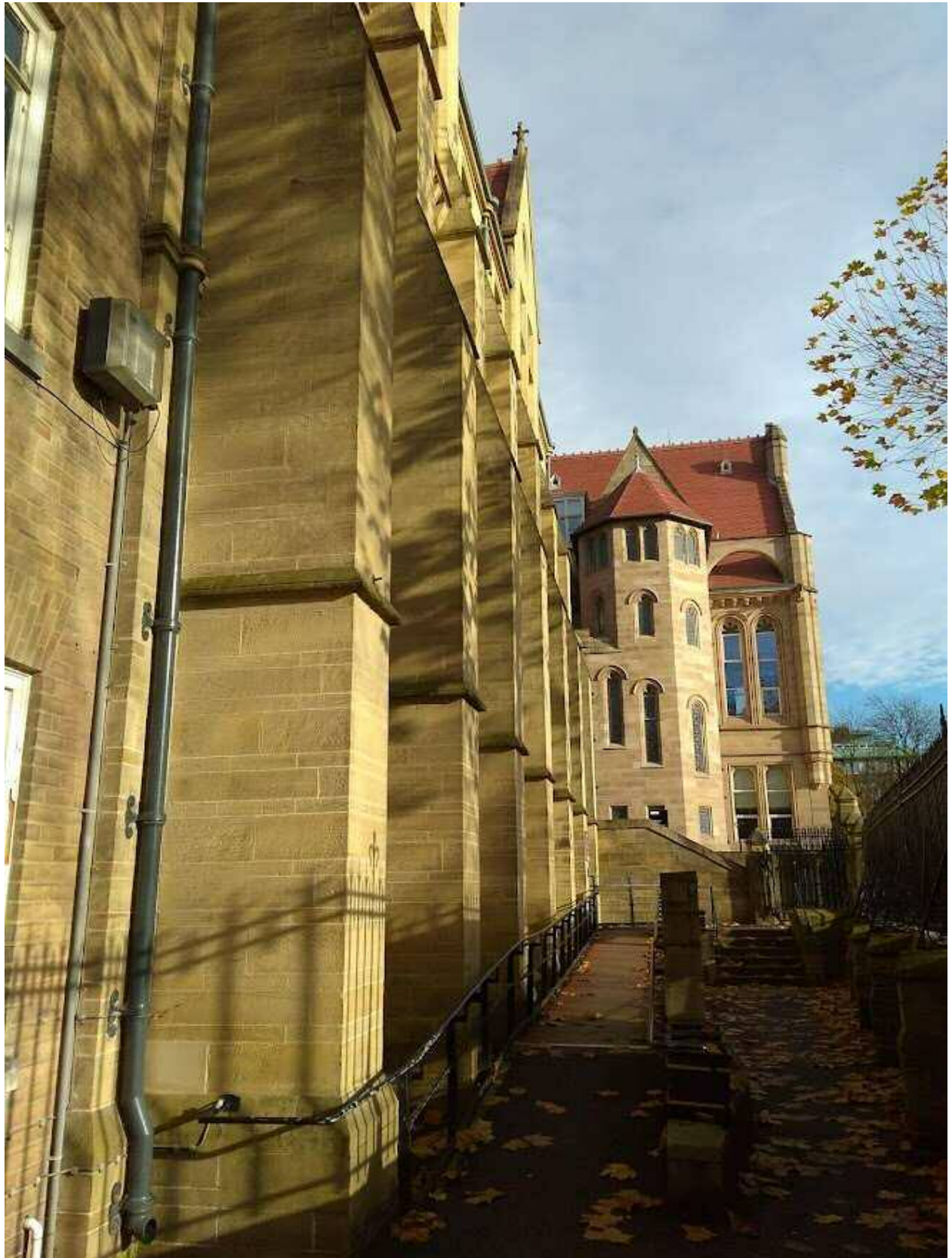
Fig 2: View up ramp on John Owens South Elevation
