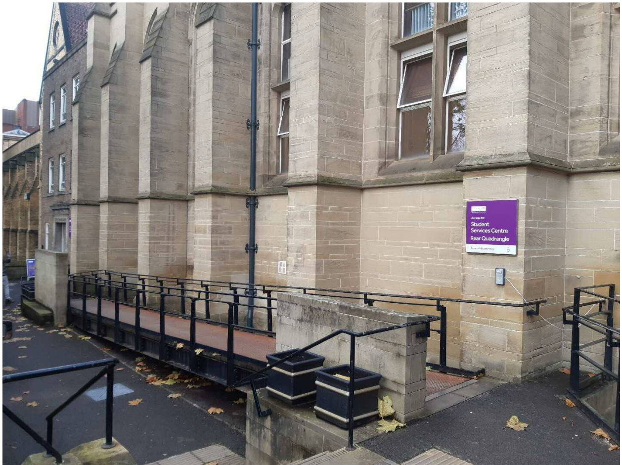
Fig 1: View of ramp down John Owens South Elevation
