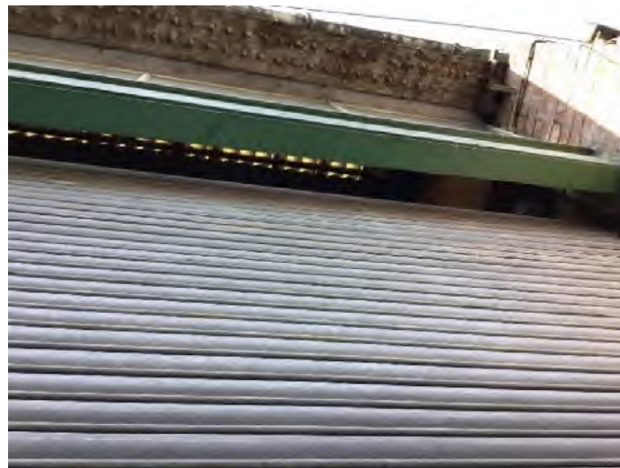
PLATE 17 SHOWING ACCESS VIA ROLLER SHUTTER DOOR
