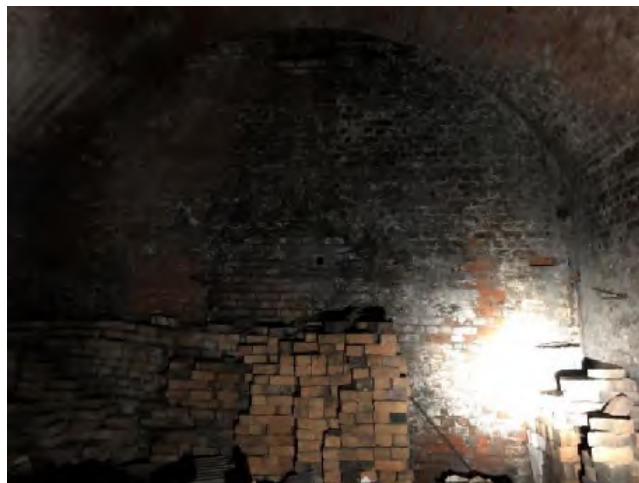
PLATE 20 SHOWING INTERNAL CHAMBER
