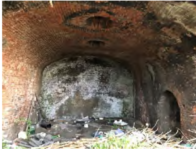
PLATE 19 SHOWING TUNNEL ENTRANCE
