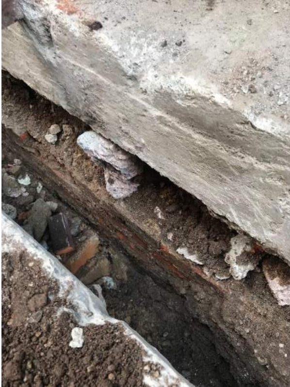
West wall of trench – facing West
