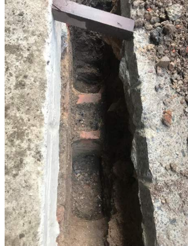
In-situ bricks encasing services – facing North
