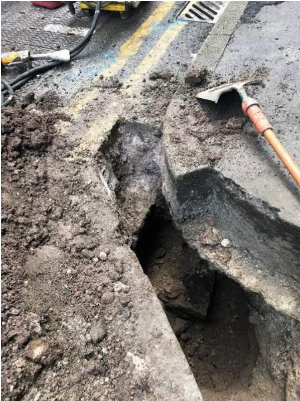
Curb to the south – facing South
