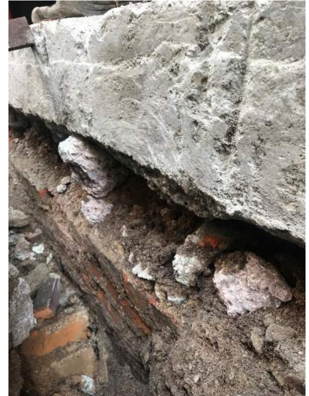
West wall of trench – facing West
