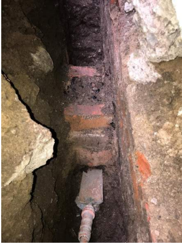
In-situ bricks encasing services – facing South
