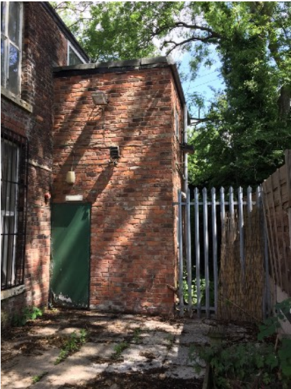
View at rear of toilet block
