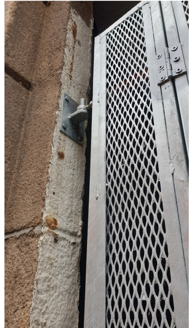
GATES/FIXING BRACKETS AS INSTALLED
