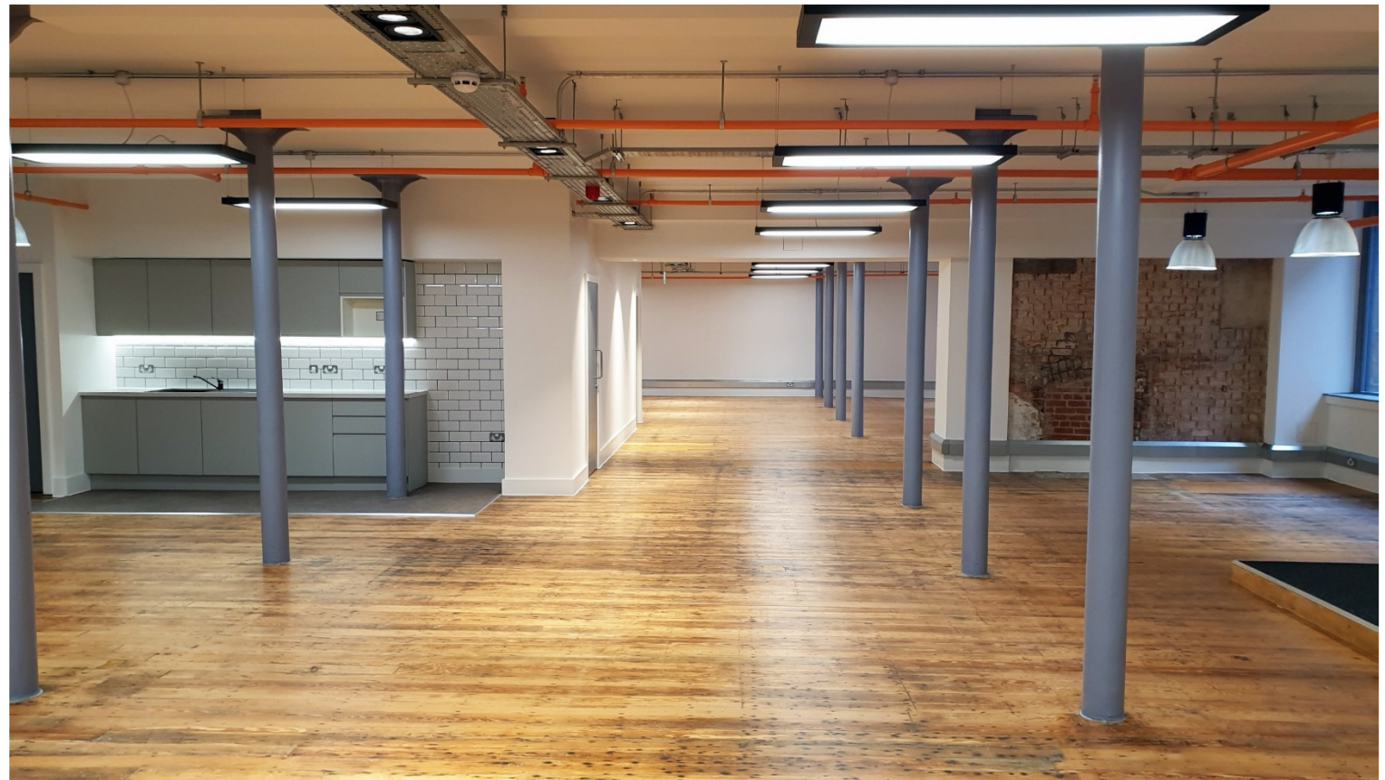
THE CURRENT CAT "A" PARTIAL IMPLEMENTATION OF THE ORIGINAL CONSENT - SHOWING OPEN PLAN AREAS EITHER SIDE OF THE CENTRAL ORIGINAL DIVISION PARTY WALL BETWEEN NUMBER 45 AND 47
