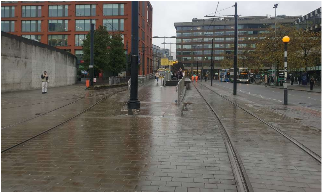
Photograph 4.4 : Metrolink Stop – Piccadilly Gardens
