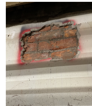
Test stripout location 2
