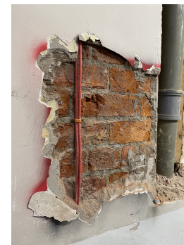
Test stripout location 1
