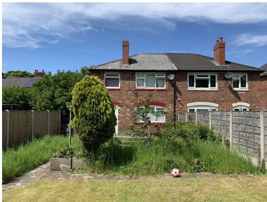
Photograph 1 Rear of 18 Cranford Avenue
