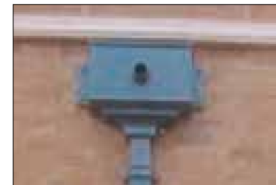
Example of hopper head fitted with spout (above) and in fabrication (right)
