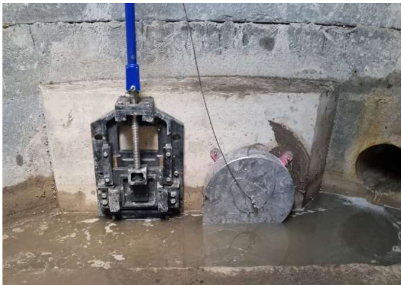
Picture 4. Hydrobrake picture
