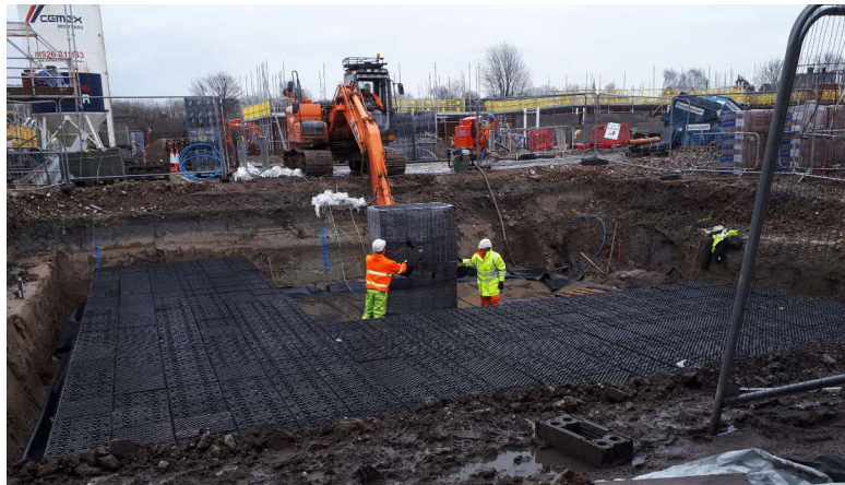
Picture 1&2. As-built attenuation tank
