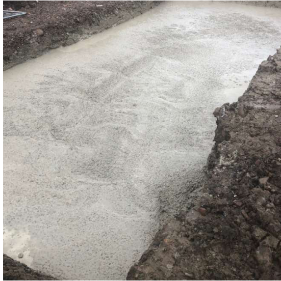
Picture 3. The concrete slab above part of attenuation tank preventing from floatation
