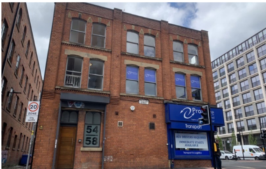
Figure 1: External appearance of the building from Newton Street
