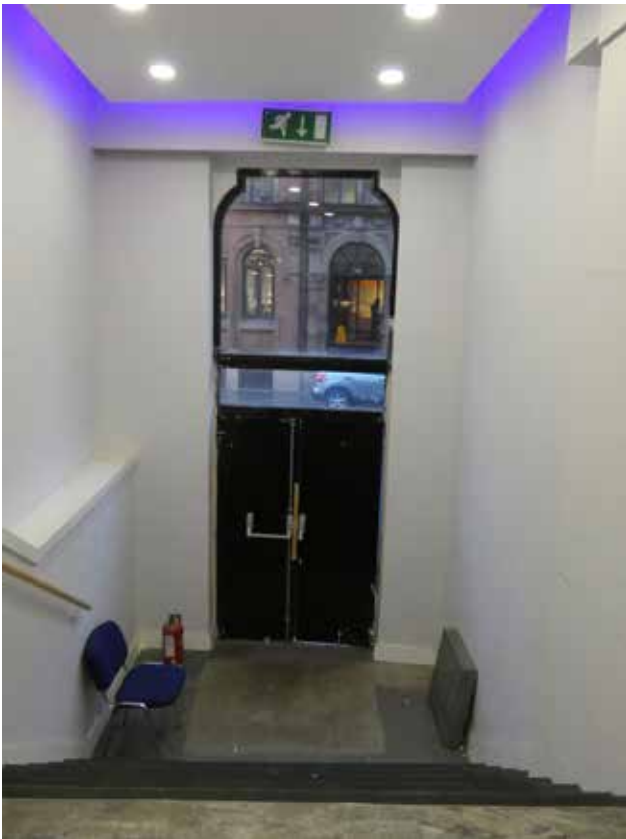
Plate 3.12 Entrance to raised ground floor through doorway at no.107 (DIA)
