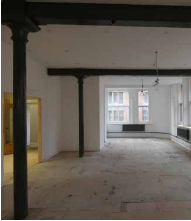
Plate 3.37 North-west corner of second floor showing exposed columns and beams, large sash windows and surface mounted cables and pipes (DIA)
