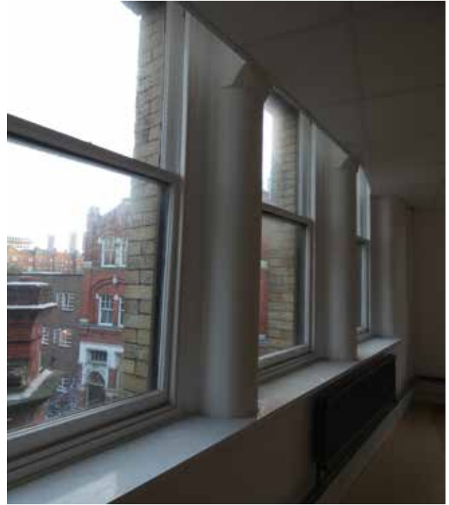
Plate 3.42 Sash windows in south elevation at second floor, partially obscured by lowered ceiling (DIA)
