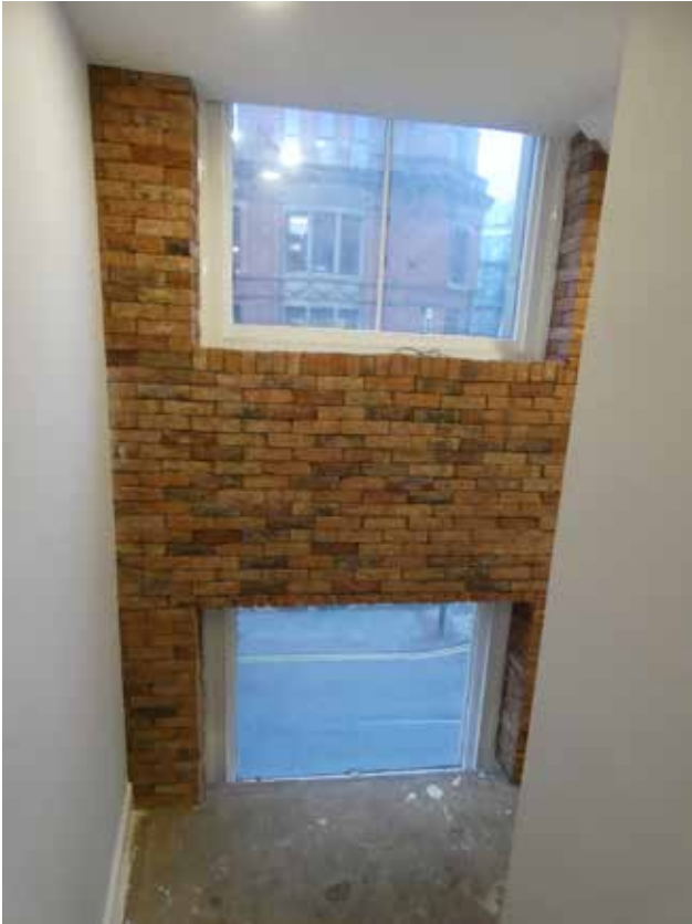
Plate 3.22 Concrete floor bisecting windows at half landing between first and second floors (DIA)
