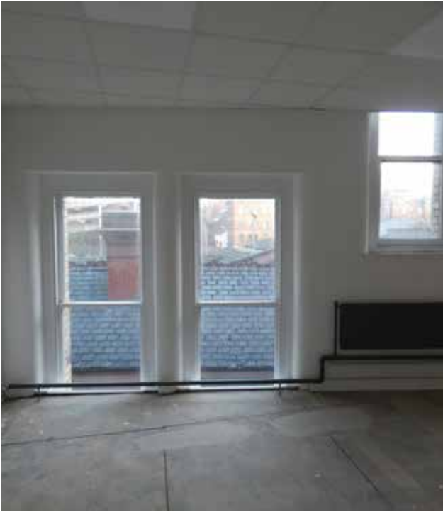
Plate 3.40 Rear windows set at half level in no.107 and partially obscured by floor plate at rear second floor (DIA)
