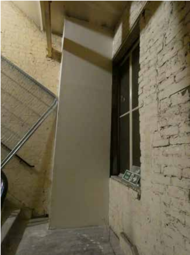
Plate 3.29 Window at first floor within secondary staircase (DIA)
