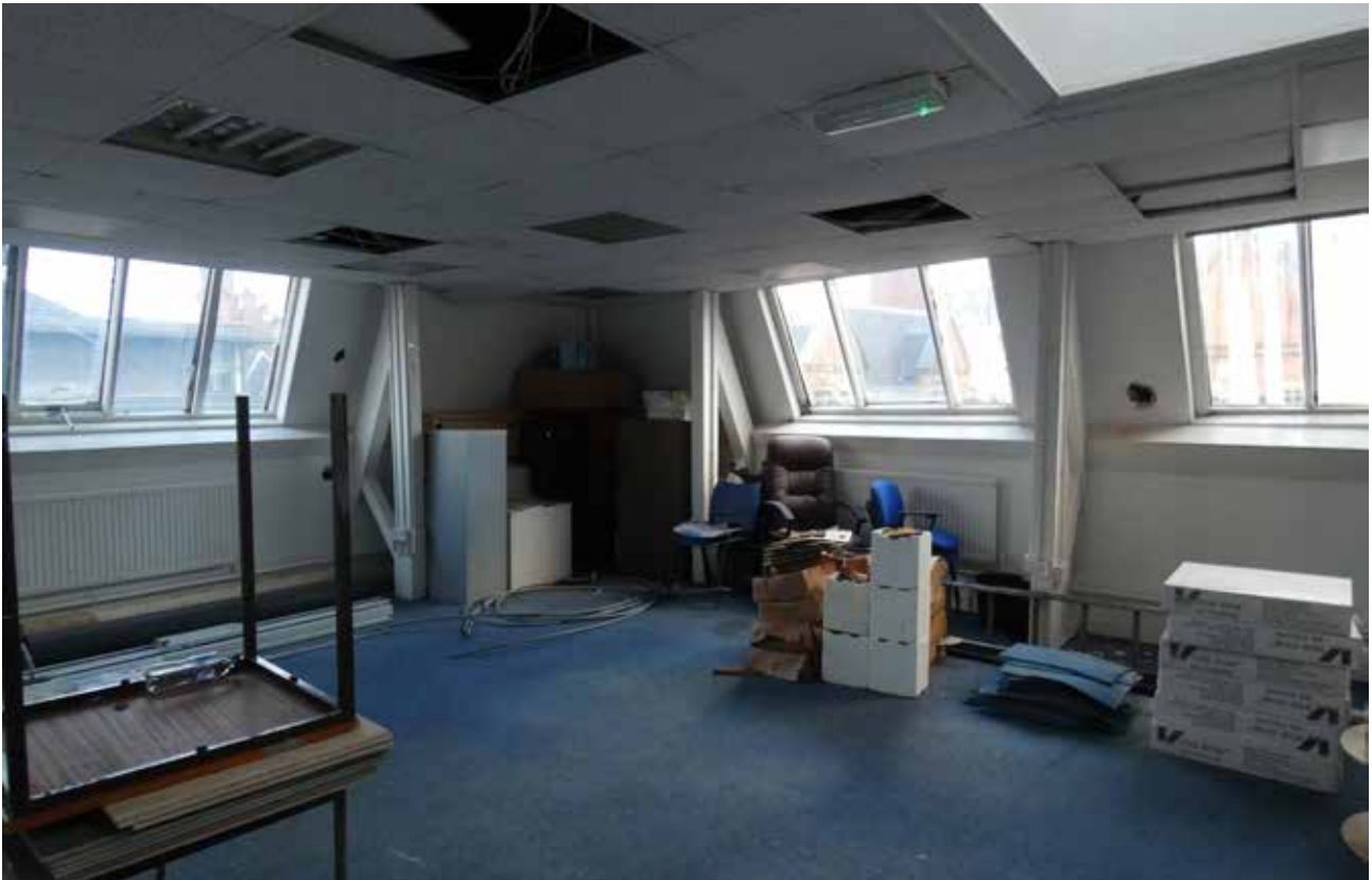
Plate 3.52 South-west corner of fourth floor showing false ceilings, exposed roof structure and roof lights (DIA)
