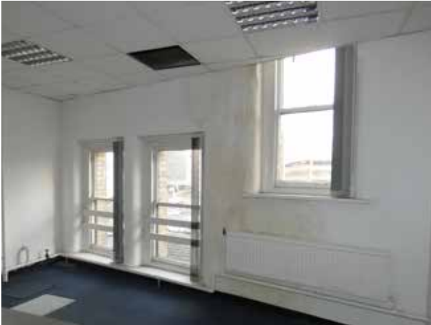
Plate 3.47 Window alignment in the centre of rear facade at third floor (DIA)
