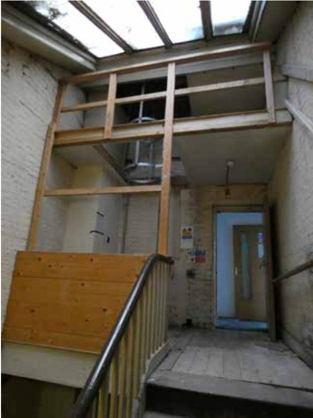
Plate 3.27 Top of secondary stair with roof light above (DIA)
