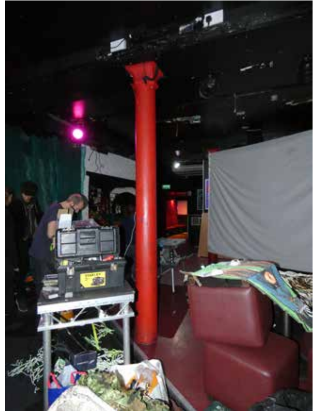
Plate 3.53b Columns in the basement club (DIA)
