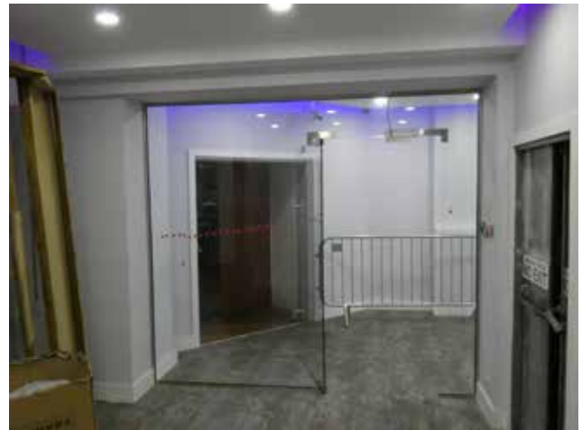
Plate 3.13 Large opening in party wall providing access from street entrance at no.107 into reception and staircore in no.105 (DIA)
