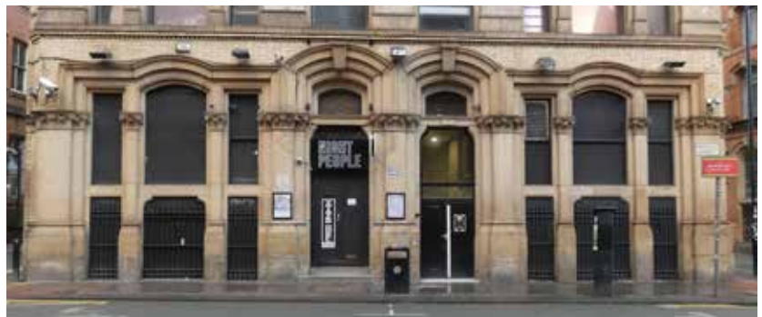
Plate 3.7 Altered entrances on Princess Street (DIA)
