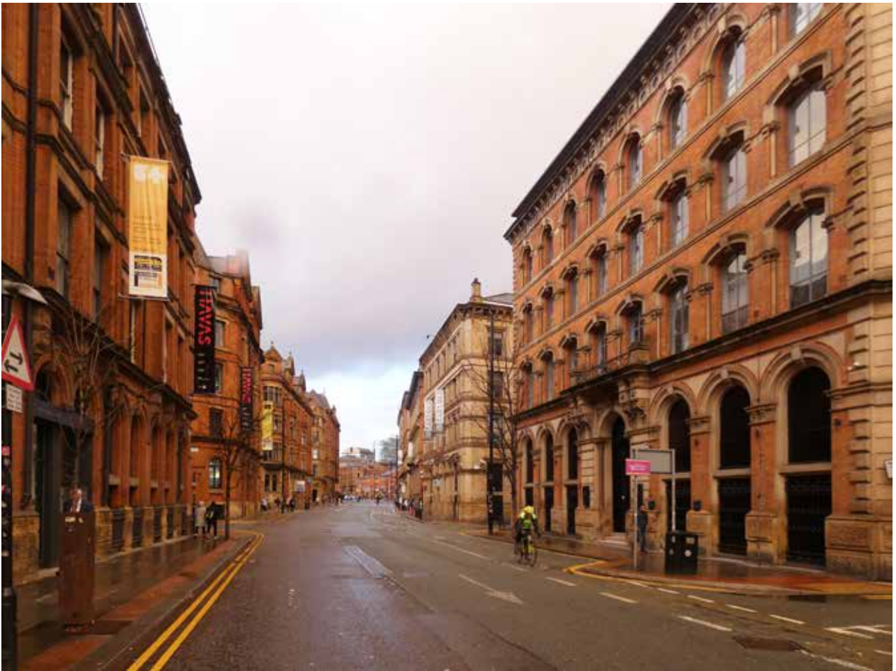
Plate 3.1 View north along Princess Street flanked by listed shipping warehouses creating an exceptional Victorian townscape (DIA)
