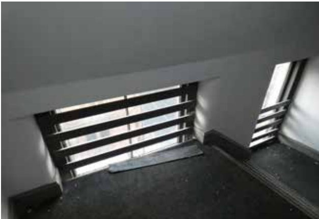
Plate 3.24 Main stair at third-fourth floor half landing, bisecting windows and skirting detailing (DIA)
