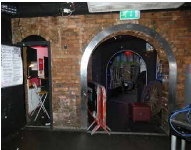
Plate 3.55 Exposed brick walls and arches at basement level (DIA)
