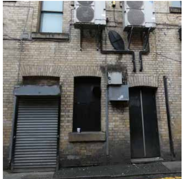
Plate 3.5 Rear facade on Abingdon Street (DIA)
