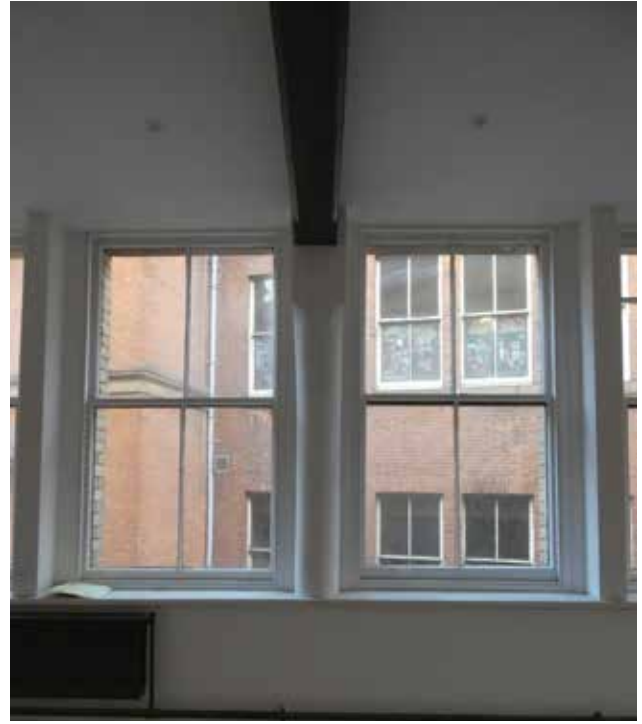
Plate 3.39 Second floor timber sash windows with roof beam and chamfered column detail (DIA)
