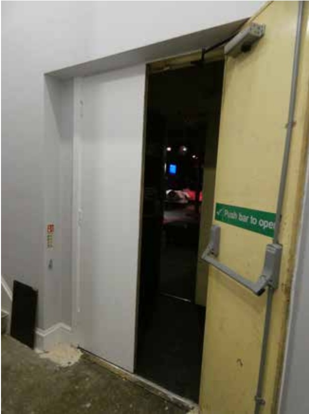
Plate 3.31 Club fire escape on to main stair at first floor (DIA)
