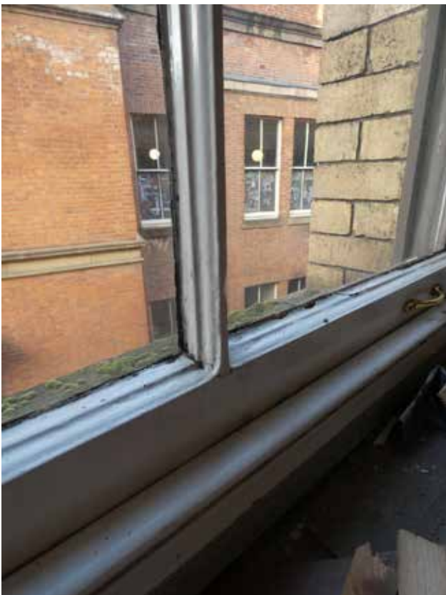
Plate 3.49a Sash window with original glazing bar (DIA)
