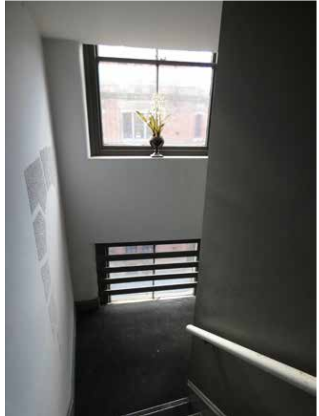
Plate 3.23 Main stair at second-third floor half landing, bisecting windows (DIA)
