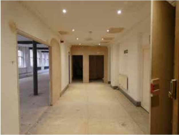
Plate 3.35 Second floor lobby currently being upgraded, WCs and services to the rear and openings in party wall to the right (DIA)
