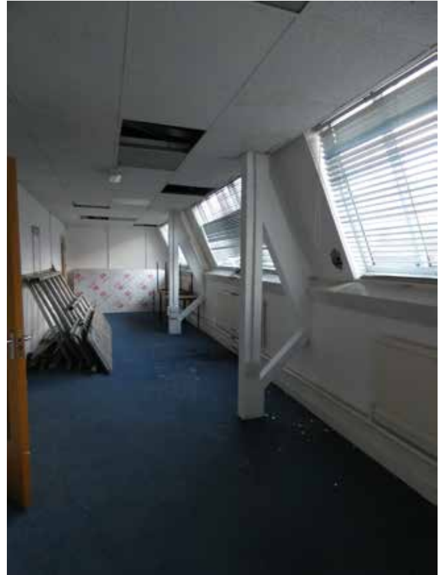
Plate 3.51 Room on north side of fourth floor adjacent to corridor, false ceiling with original timbers above showing lathe scars (DIA)
