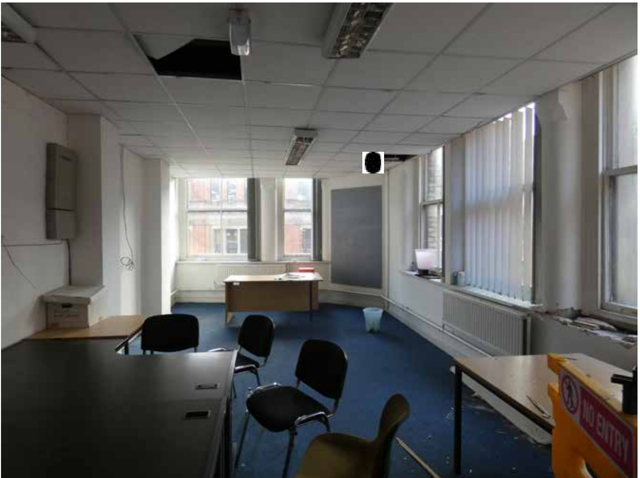
Plate 3.44 Third floor north-west corner (DIA)
