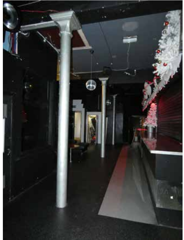
Plate 3.32 Iron columns in first club area in no.105 (DIA)
