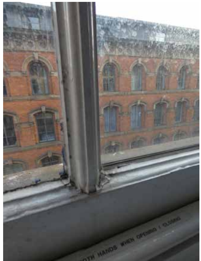
Plate 3.49b Sash window with splice repair (DIA)
