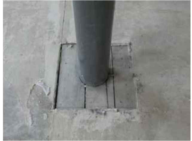
Plate 3.36a Original timbers around columns at second floor (DIA)
