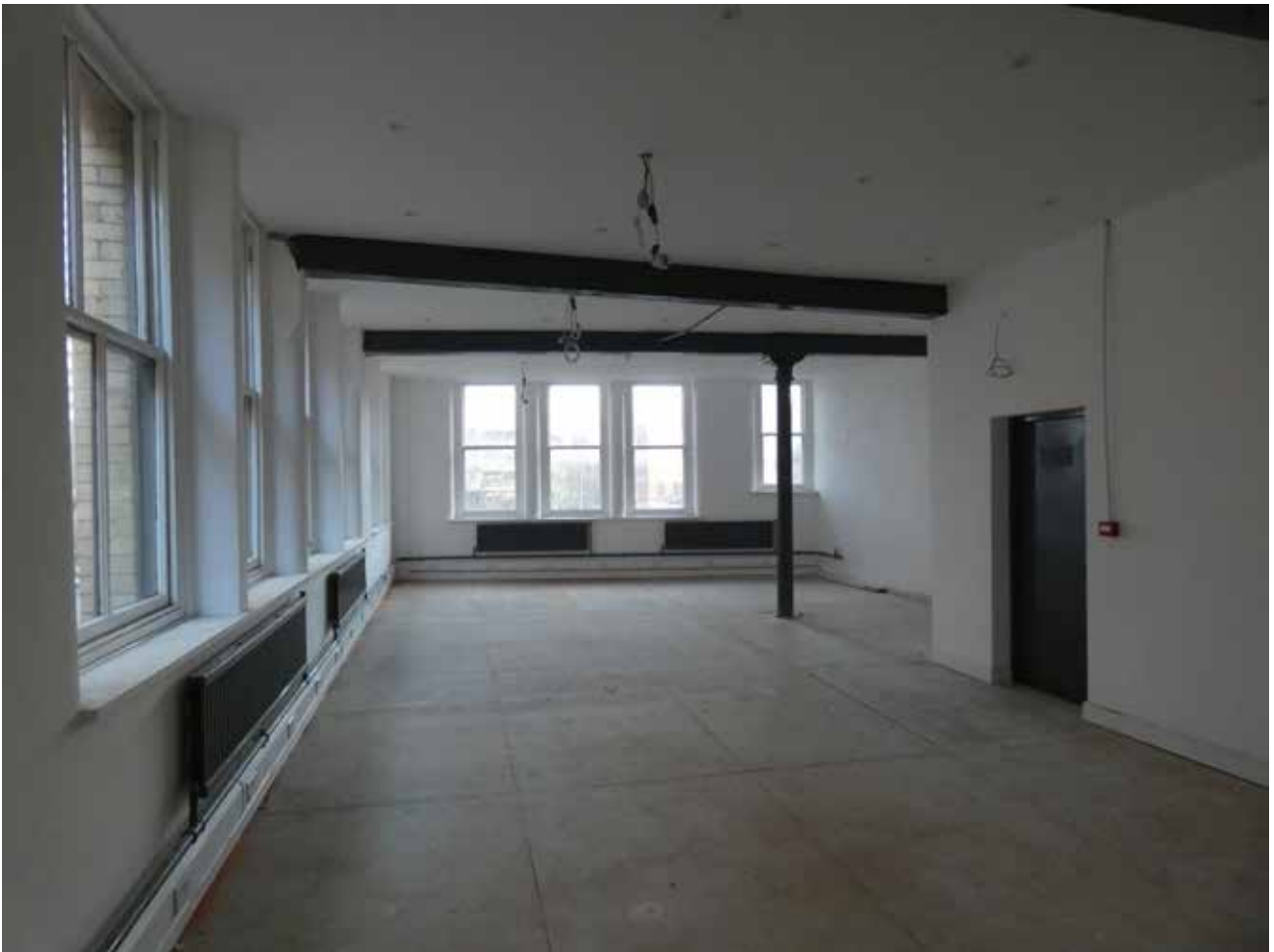
Plate 3.38 Rear of northern side of second floor (DIA)
