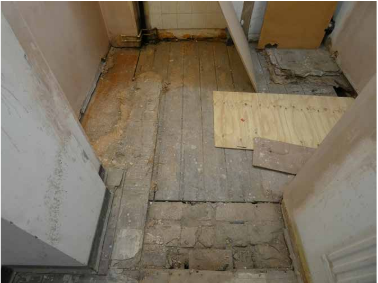
Plate 3.36b Original brick flooring in WC core at second floor (DIA)
