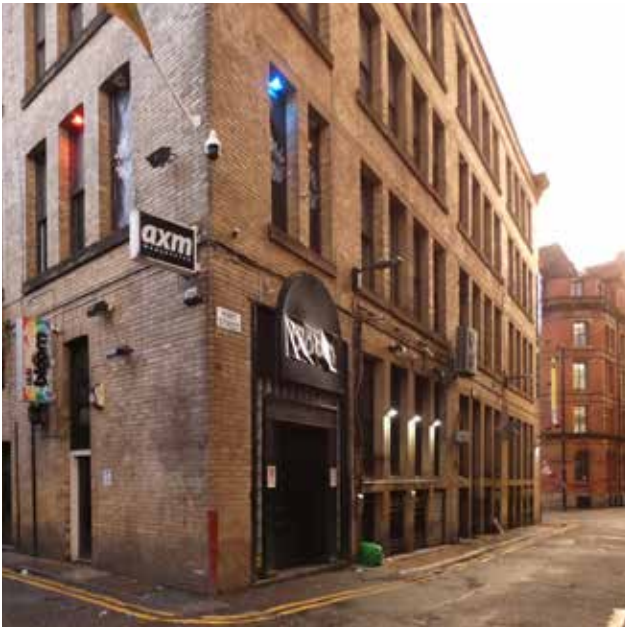
Plate 3.4 Side elevation to Hart Street with double height service access opening and more restrained character to this and rear facade (DIA)
