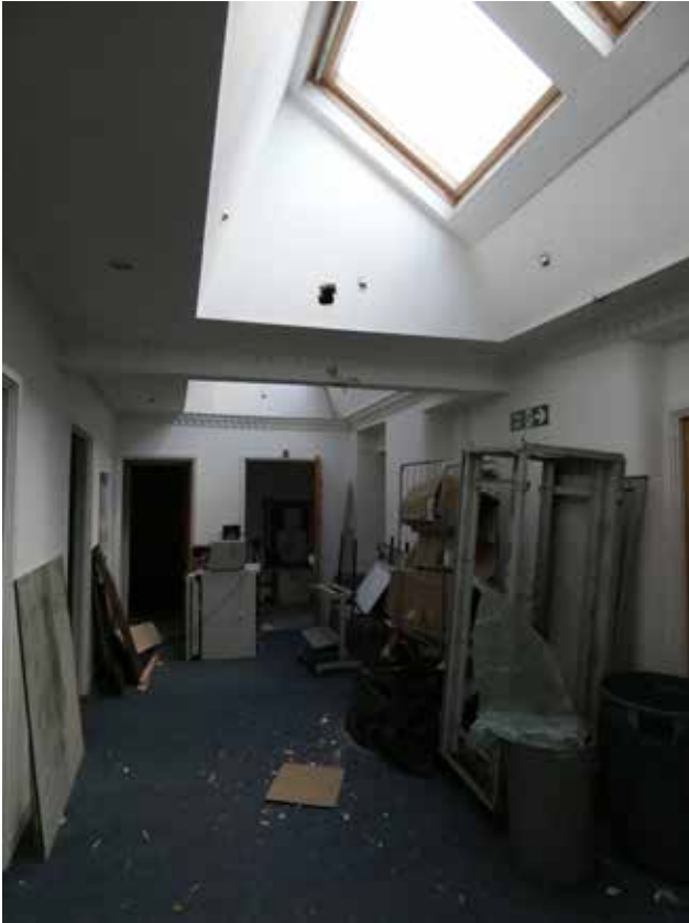
Plate 3.50 Fourth floor central lobby with modern partitions, decorative features and rooflights and openings in the party wall to the right (DIA)
