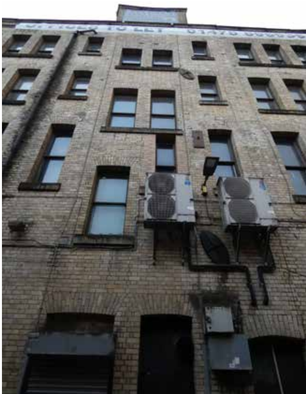
Plate 3.10 Offset windows to rear elevation and roof tower above (DIA)
