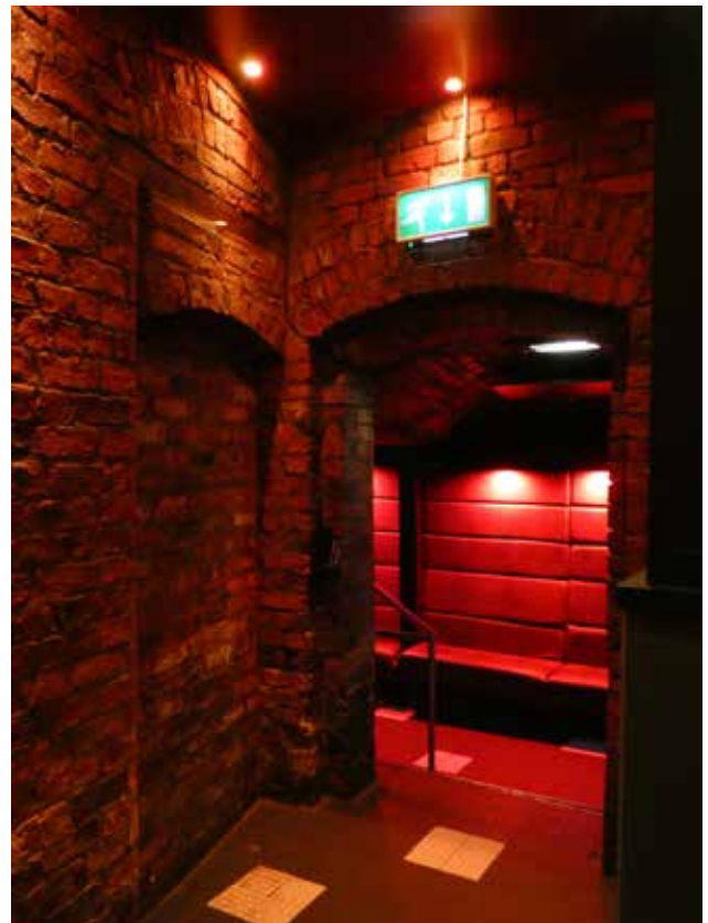
Plate 3.54b Vaulted ceilings at basement level under former loading bay (DIA)
