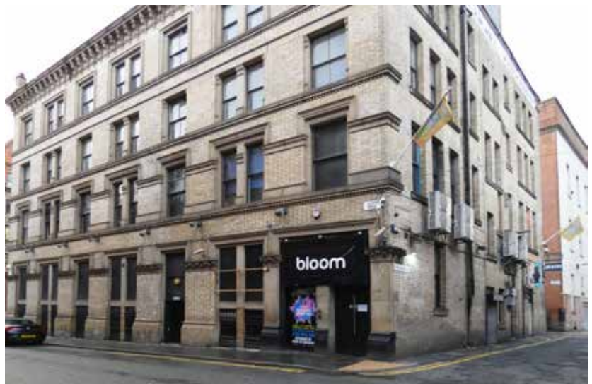
Plate 3.8 Bloom Street elevation and former loading bay access (DIA)
