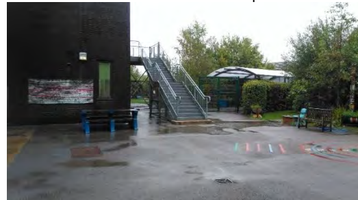
View north from the southern tip of the site
