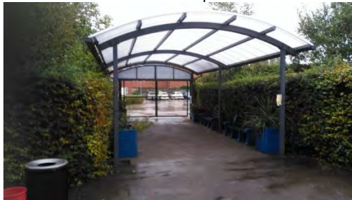
View west towards the site entrance
