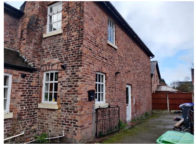
The north elevation
