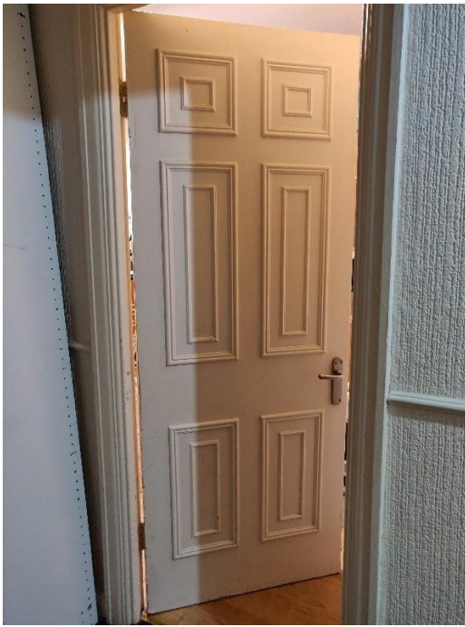
Door in ground floor hallway
