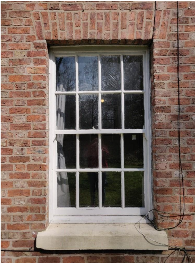
Replacement sash window to south elevation
