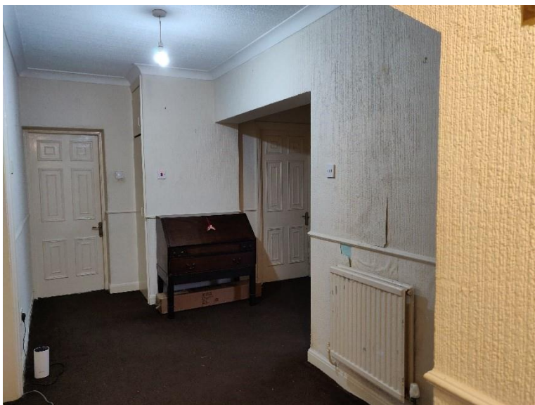
Ground floor hallway
