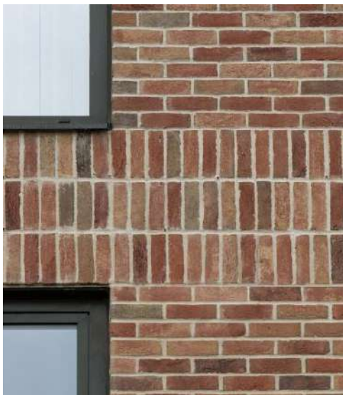
Vertical stack bond brick detail
