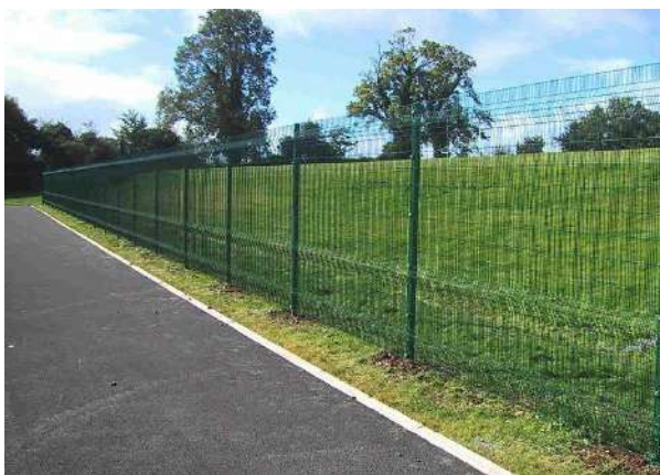
Palladin fencing to be installed
