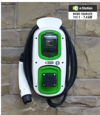
Standard Mode 3 7.4kW EV Charger
